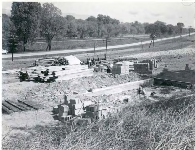
An unusual sight, caused by the current scarcity of lumber. The owner of this property, who is building his own home, has set up a sawmill, visible in the picture, and sawed out his building lumber on the site from logs he had purchased. He is using oak lumber, and it will not have to be air-dried before use because the logs had been cut about 2 years before he sawed them. Near Whitman, Minn. April 1946.
