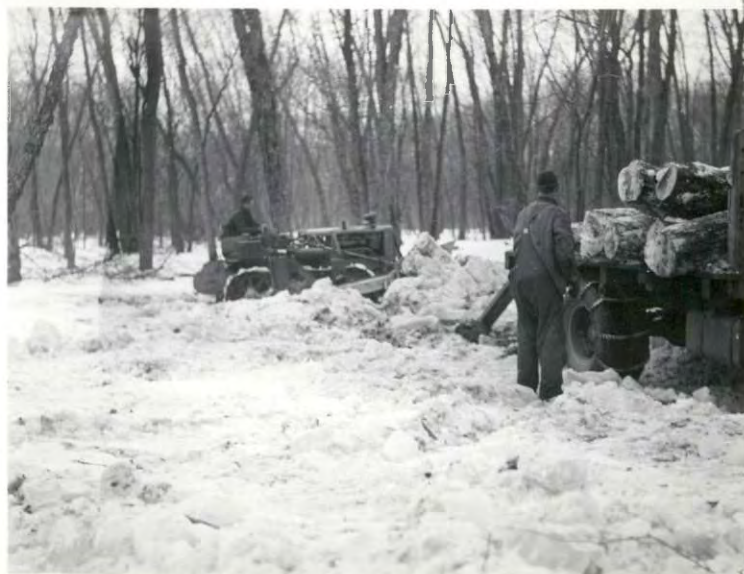
Bucking logs out of ice with "cat". Black River bottoms. February 25, 1946.
