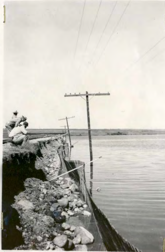
Soo Line grade damage at Greene Crossing
