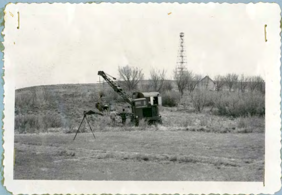
Preparing to excavate basement for Res. #2. Hanson Crane being used.
