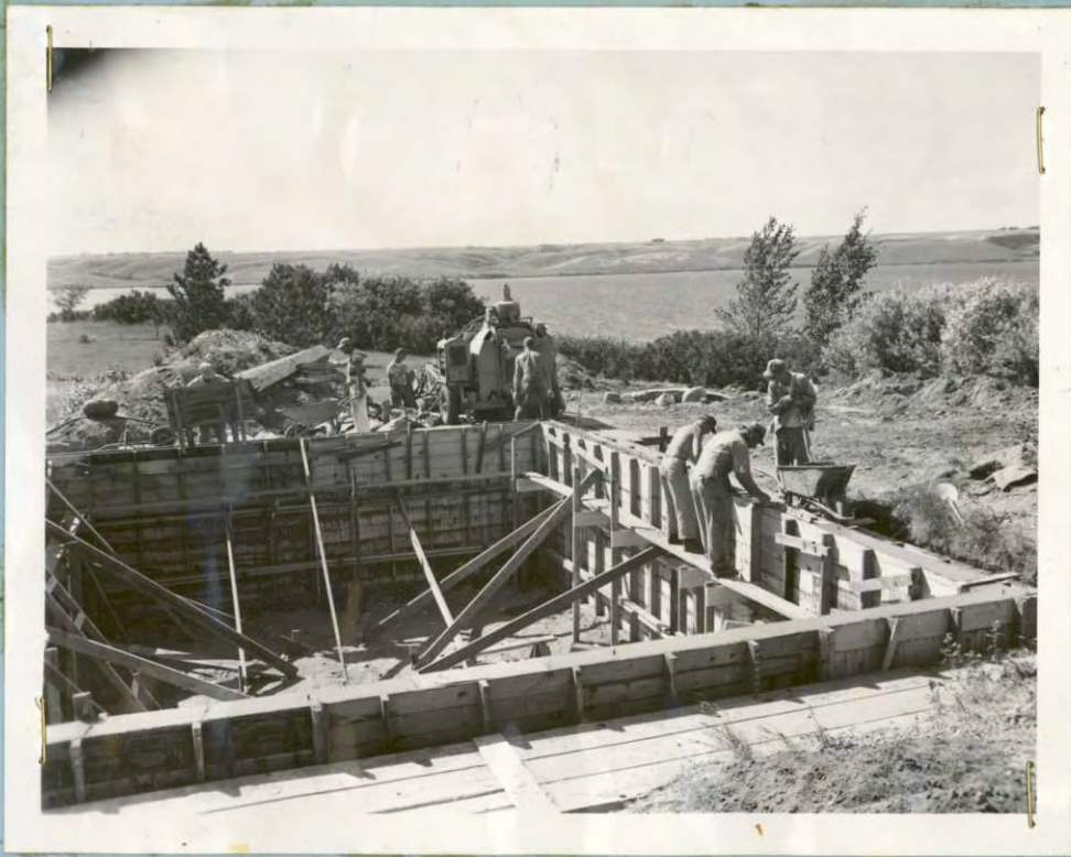
Pouring basement wall for Res. #2. Man leaning on shovel is no longer with us.
