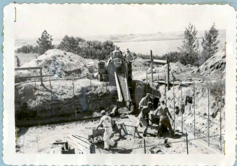
Pouring foundation footing for Res. #2 (Clerk's residence) which will be moved in September.
