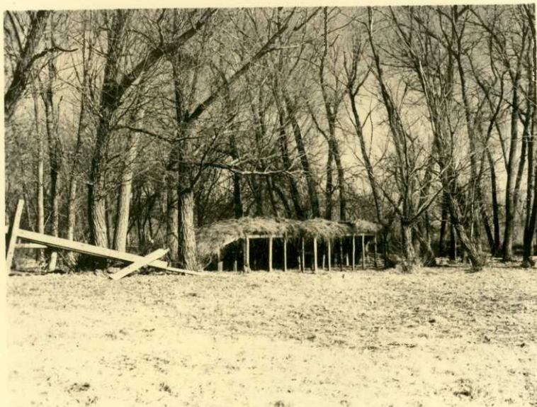
Same shelter as shown in above photograph but it has been completed by covering with hay and binding down with salvaged wire.
