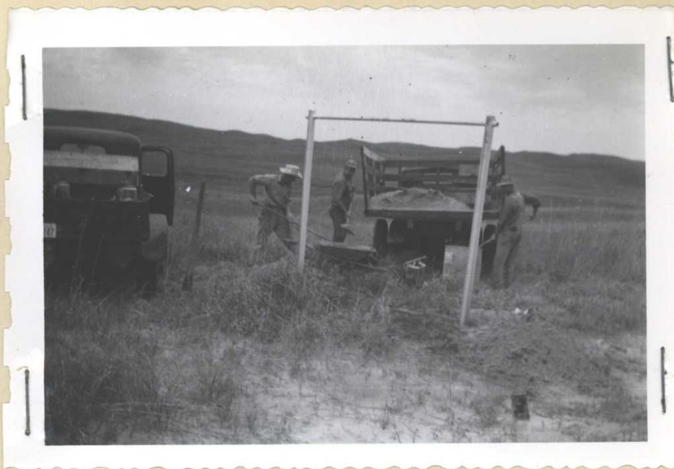
Clerk Wilson and Maintenance men Swanson and Hauge erecting pipe sign frame. Posts are set in concrete, and concrete anchor chains are also attached to the sign to prevent wind damage.
