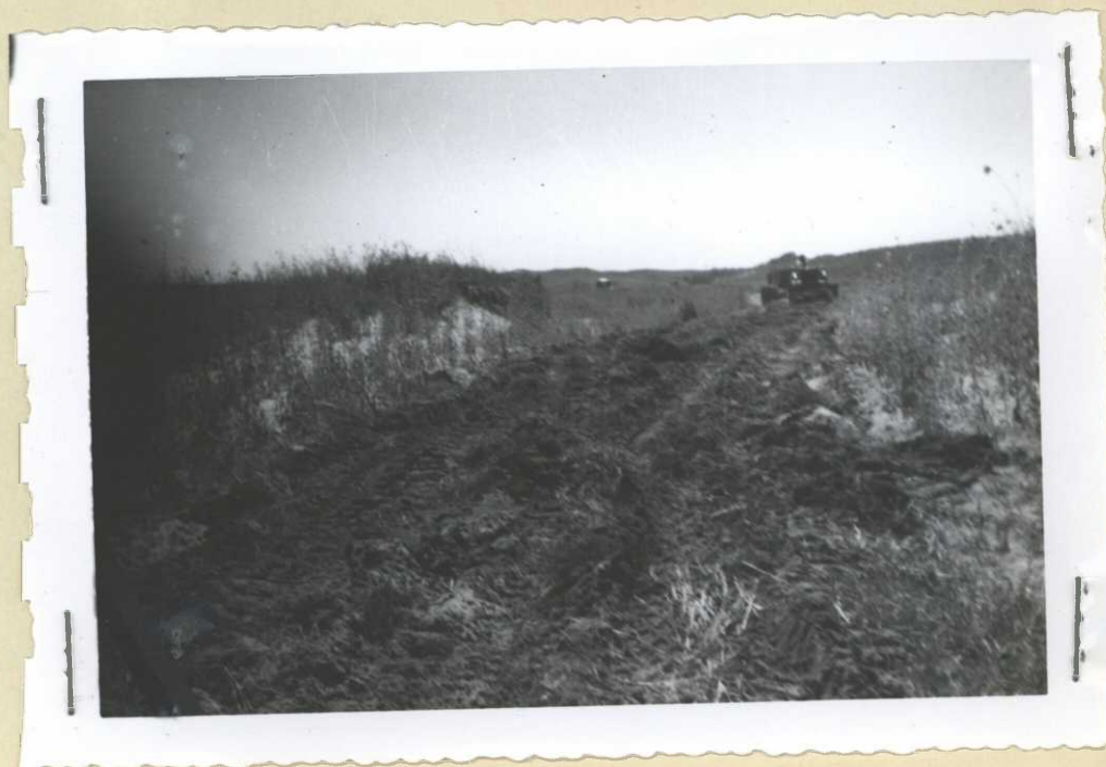
Cuts made through impassable sand hills are leveled and 'paved' with sod and black dirt from adjacent meadowland. Td-9 and 5yard scraper used for this work. These cuts are on the Hackberry-Dewey Canal and along the north side of Dewey Lake.
