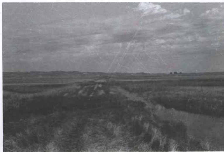
The roadfill between North Marsh and Middle Marsh Lakes is no longer passable at the east end. The fill is also under water at several other spots farther west. The Marsh Lakes basin does not drain with present water levels.
