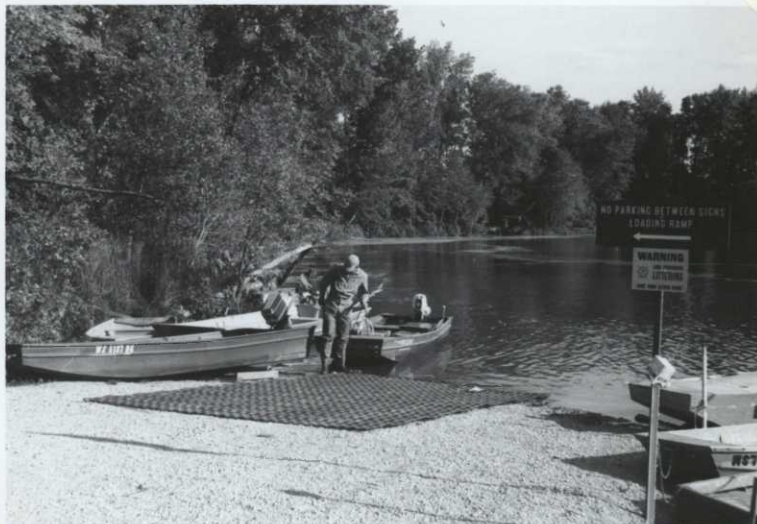
Aircraft landing mat installed on ramp at Bertom lake landing. We use about 21 mats and weld them together so they won't be stolen. The mats extend out under the water as far as the trailer will be backed and do an excellent job of keeping the ramps from being torn up.
