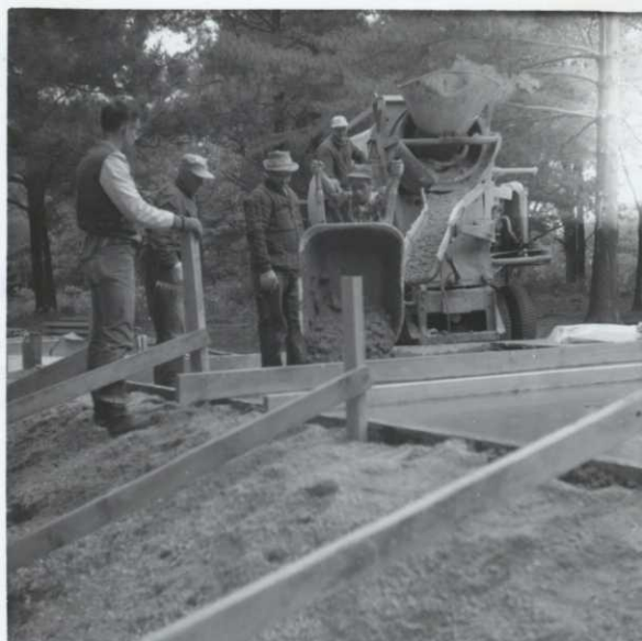
Pouring foundation for new district warehouse.
