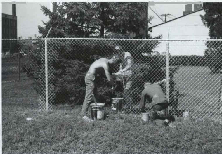
Painting chain link fence with rollers on each side-- a very efficient operation
