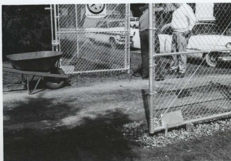
crushed rock placed to prevent weed growth under fence
