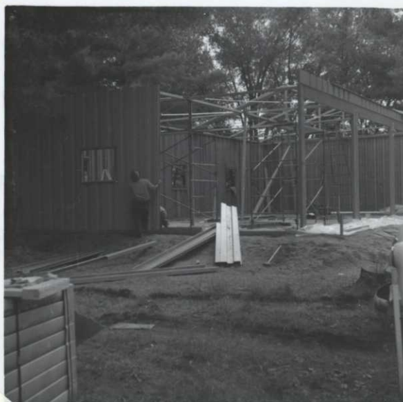
Up go the sides of the 28 x 56 Armco metal building.
