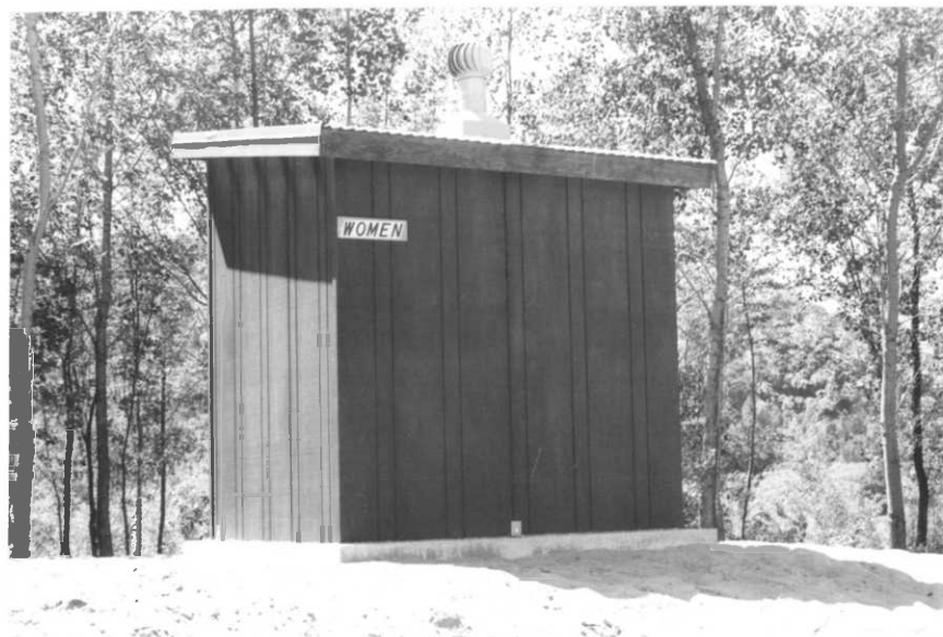
After: a new building placed over a new concrete holding tank. R-5-71-16 MAK
