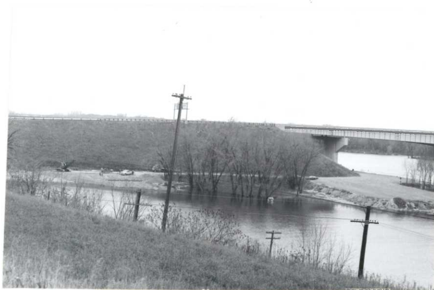
The Minnesota Highway Department had completed hauling of fill-base for access site. 830 cu yds of gravel were used on entrance road and parking area. R-10-71-4 MAK
