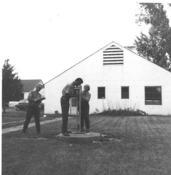
Janet Smith, the second of two Biological Aides, levels the steel supports that will brace the flag pole. Larry Nelson takes needed measurements while one of the summer NYC's record the measurements for further reference. Holes were drilled into the old wood base, saturated with fuel oil, and burned. Continual burning removed enough of the wood to allow steel supports to be erected and cemented into place. B-279-2 1971 Leinecke
