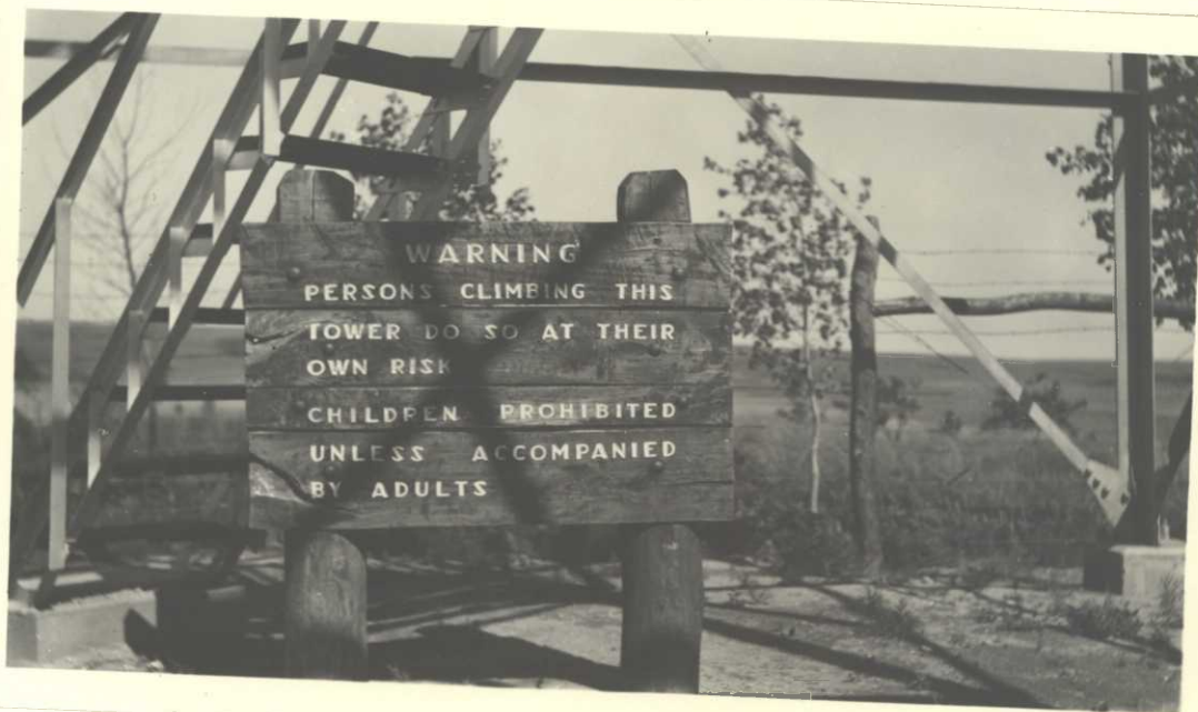
The warning sign at the tower.
