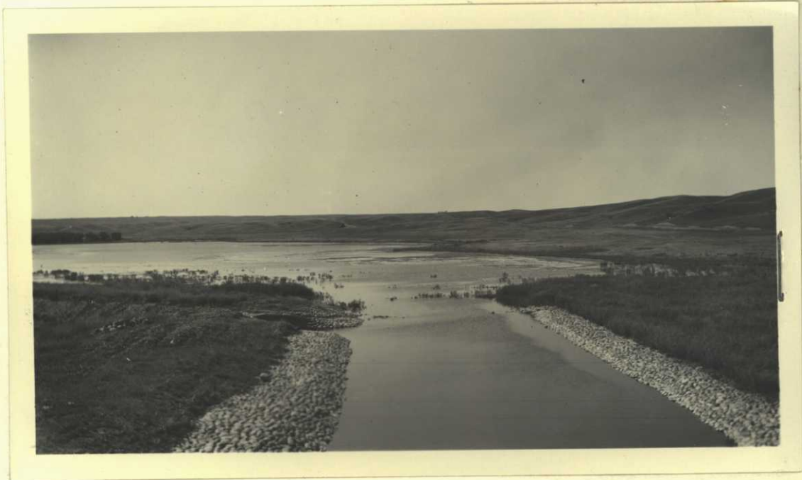
Looking over Pond A from the control of Dam 83.
