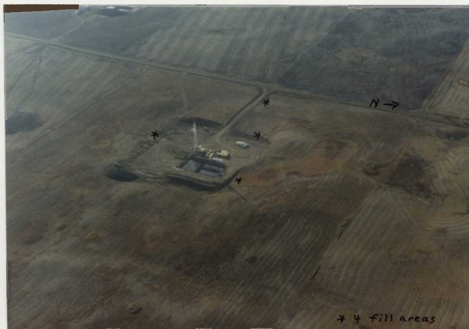
Figure 18. Oil well pad site partly filling four wetlands on Ward 267x. (11/88. RA 30A-88-21)
