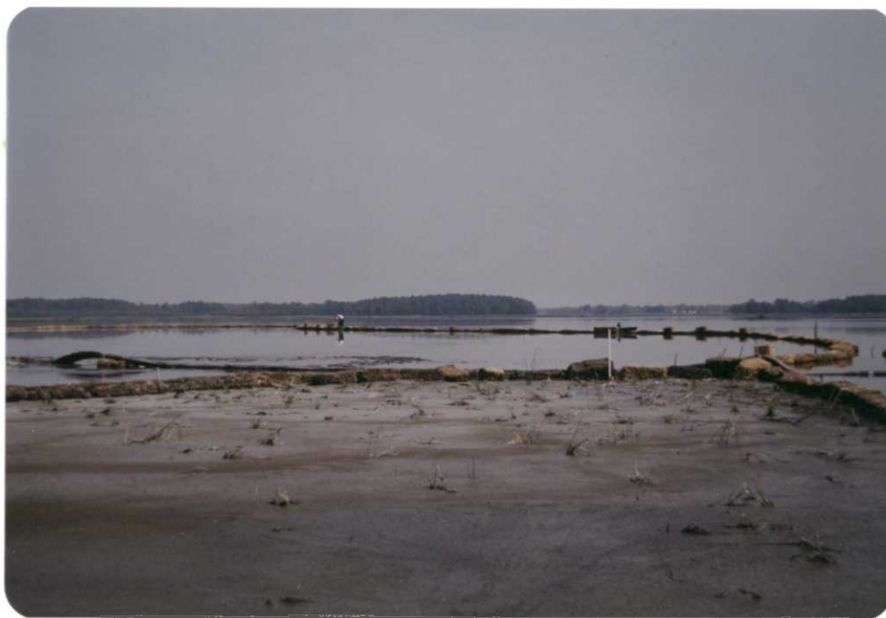
Pumping dredge material into straw bale containment barrier
