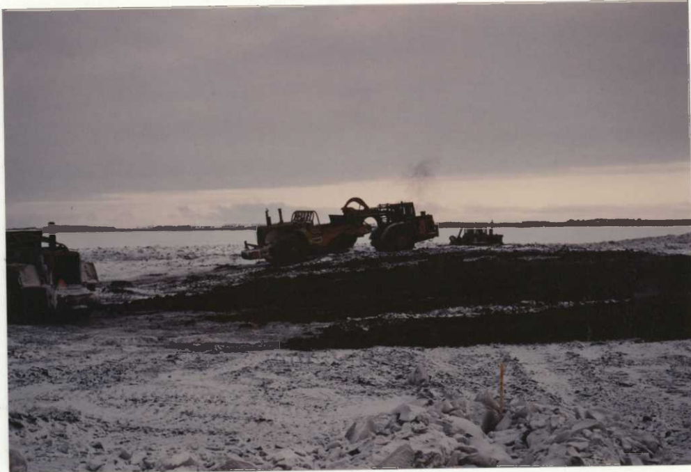
Photo # 3. Earth mowers hauling fill to DU island. Bulldozer is scraping ice away from the lake bottom. 1/87 DAL
