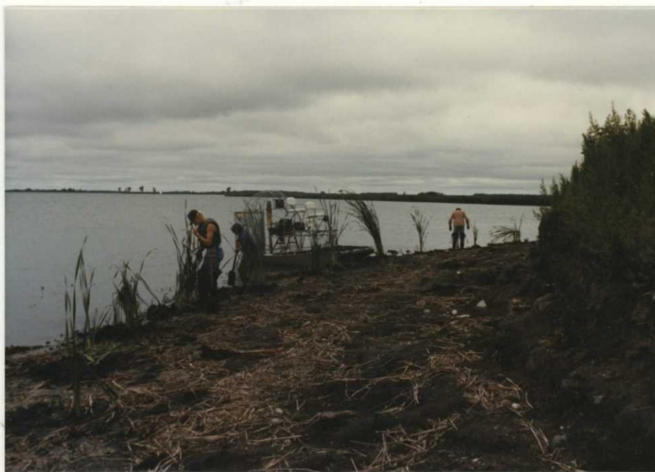
Photo # 5. Crew transplanting cattails on island shoreline. This second attempt failed to establish an emergent buffer. 7/87 RAH
