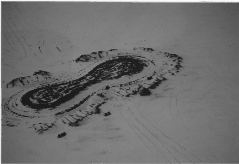
Photo # 2. Hour-glass shape of DU island minimizes wave action, adds shoreline, and has a natural appearance. 3/87 DAL
