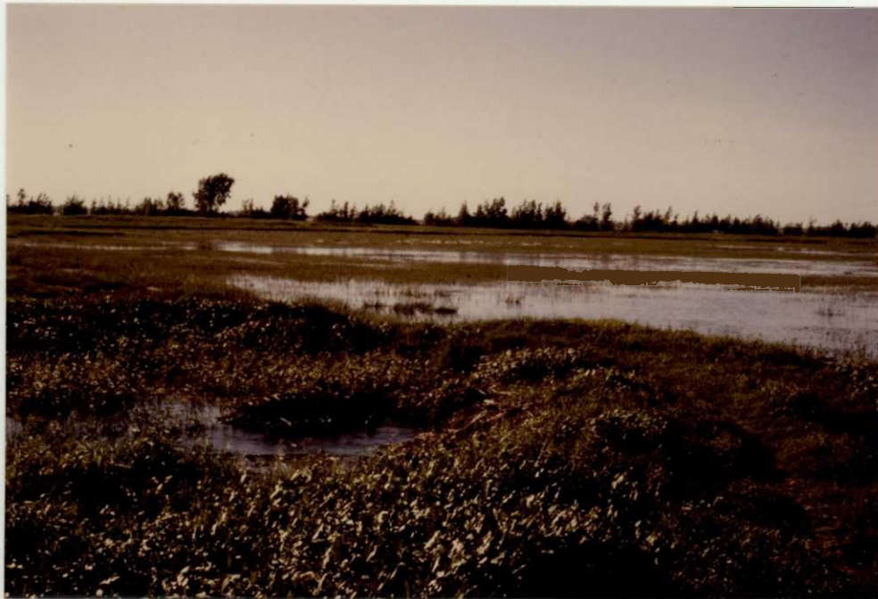
Photo # 10. Outlet of Traynor Lake: note flooded shorelines and water rushing from culvert under Service road.
