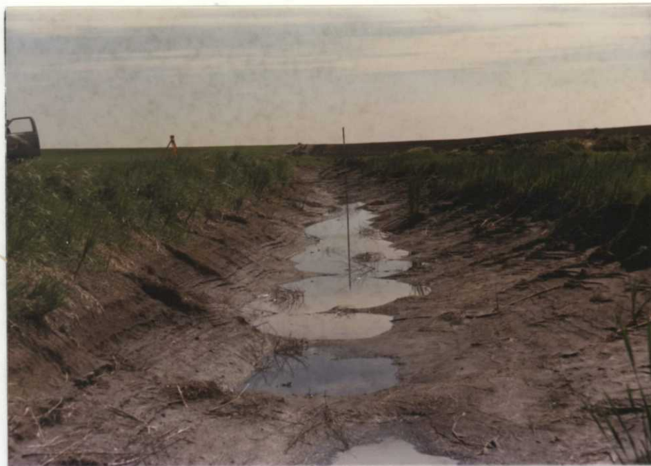
Photo # 8. One hundred thirty nine easement cases were opened in 1987, seventy-two consisted of scraper or loader-type ditches. This keeps the enforcement staff busy. RWS
