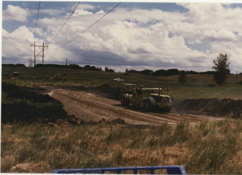
Eighty wetland restoration projects were completed on district WPA's in 1987. This dam (and plumbing) under construction on the Arneson WPA, Becker County, was paid for by two local sportsmens clubs. LH 7/87.
