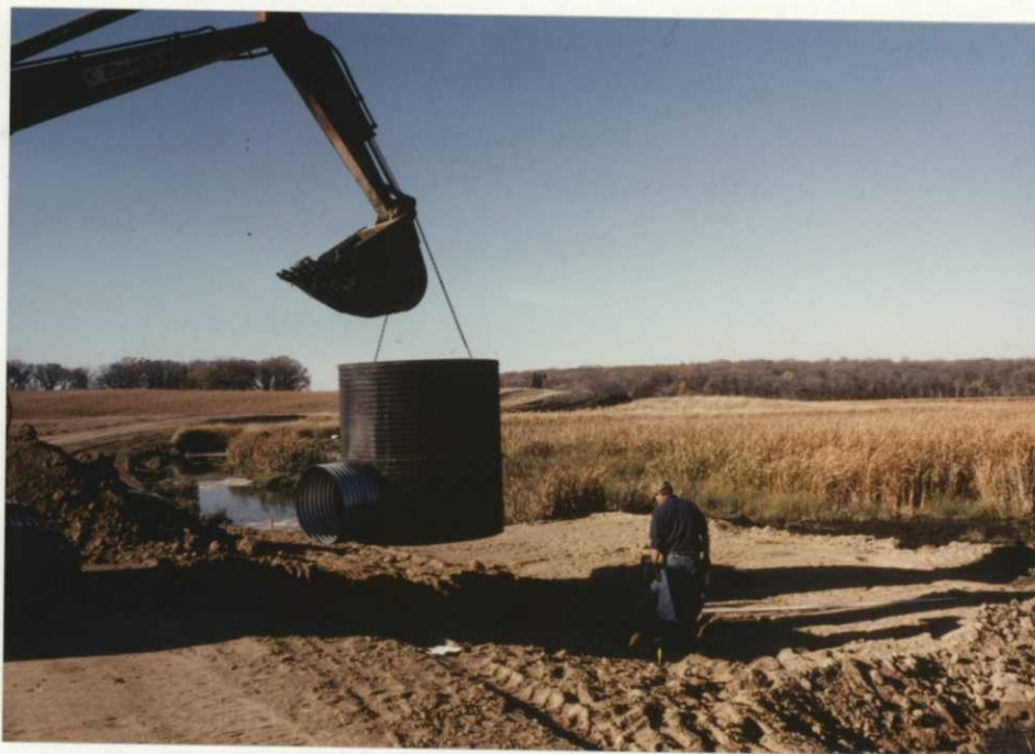
Installation of Rotary Carp Screen on Nicholson WPA (OT-88), Otter Tail County. EW 1199
