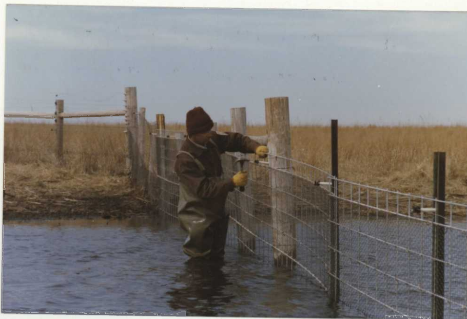
"Water wings" are constructed using 14-foot cattle panels with one-inch hex mesh attached. The separate sections of the wing allow for easy installation and removal after the nesting season. Sections can be added if water levels drop. WS 4/88
