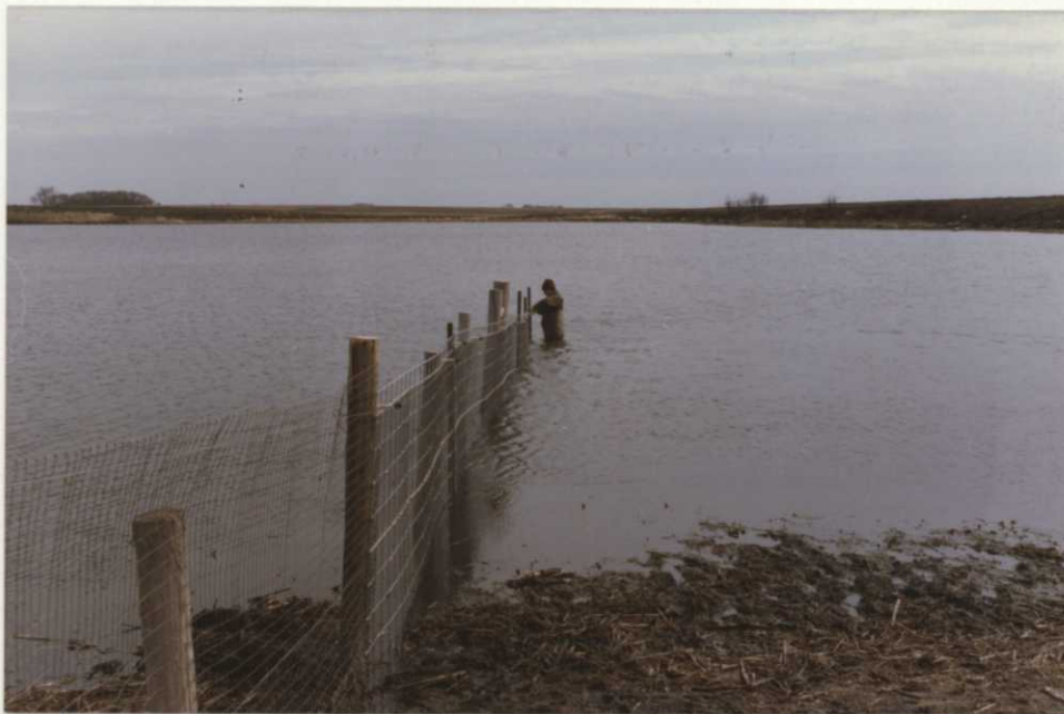
Where predator fences intercept wetlands "water wings" are constructed to discourage predators from swimming around the ends of the fence. One charged wire extends the entire length of the wing. WS 4/88
