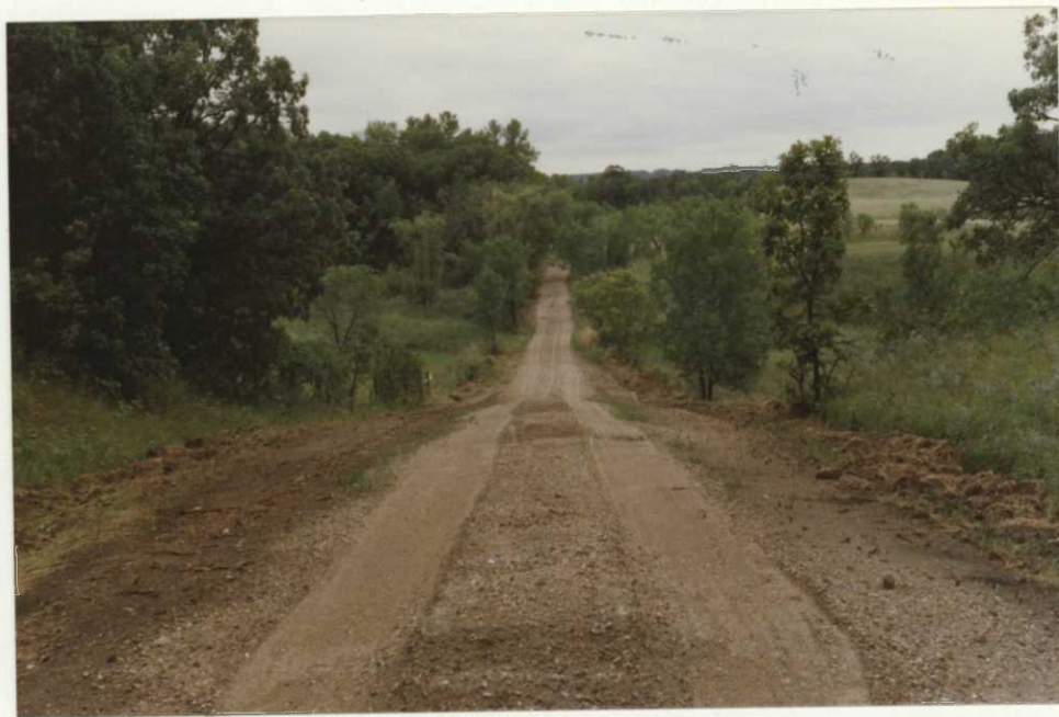
The same trail on Banke Slough WPA after scalping sod and brush with a road patrol followed by a top dressing of class five crushed gravel. CV 7/88
