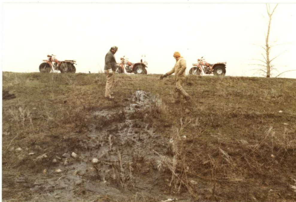
Photo 50. Inspecting a leak discovered in Bonehill NWR dam, 4/84 - LDW
