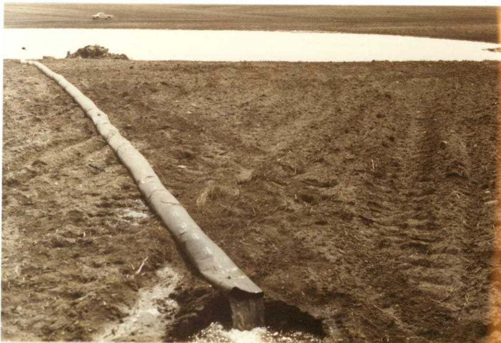
Photo 30. Collapsible pipe heading over the hill to facilitate drainage from floating pump, 4/84 - JWJ.
