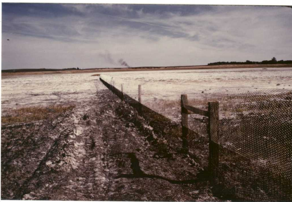
Photo 33. Initial construction of electric fence at Bovey WPA using 1" mesh buried one foot in the soil and to a height of 5 feet. Electric wires will be placed directly in front and on top, 10/84 - RAH.
