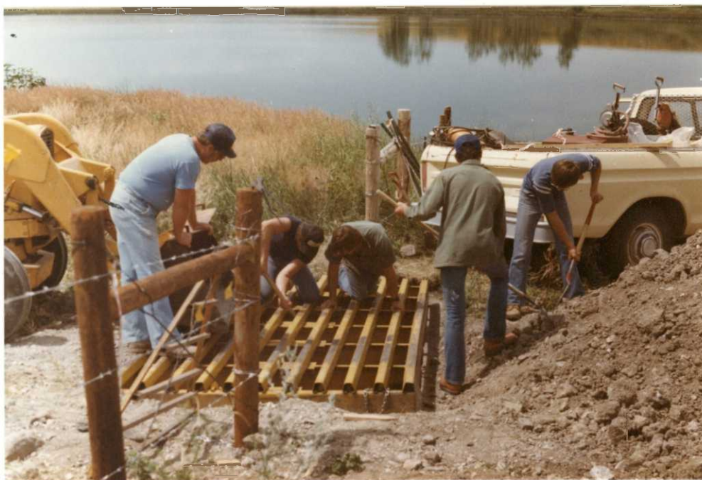
Photo 8. YCC installing cattle guard at Mundt Lake WPA, 6/84-JWJ.
