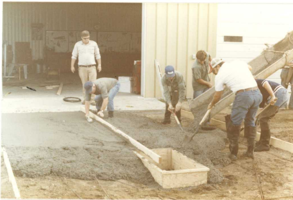
Photo 44. Construction of vehicle wash rack at shop site, 7/84 - JWJ
