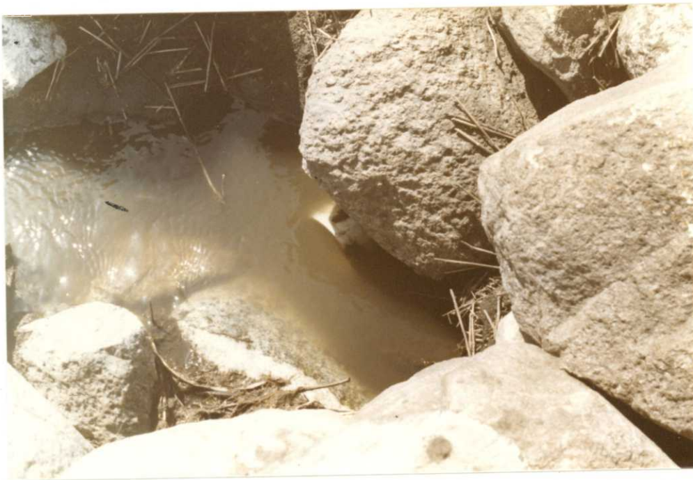
Photo 26. A closer look at the same rock pile shows the tile drain exit which is efficiently draining the wetland, 5/84 - RAH.
