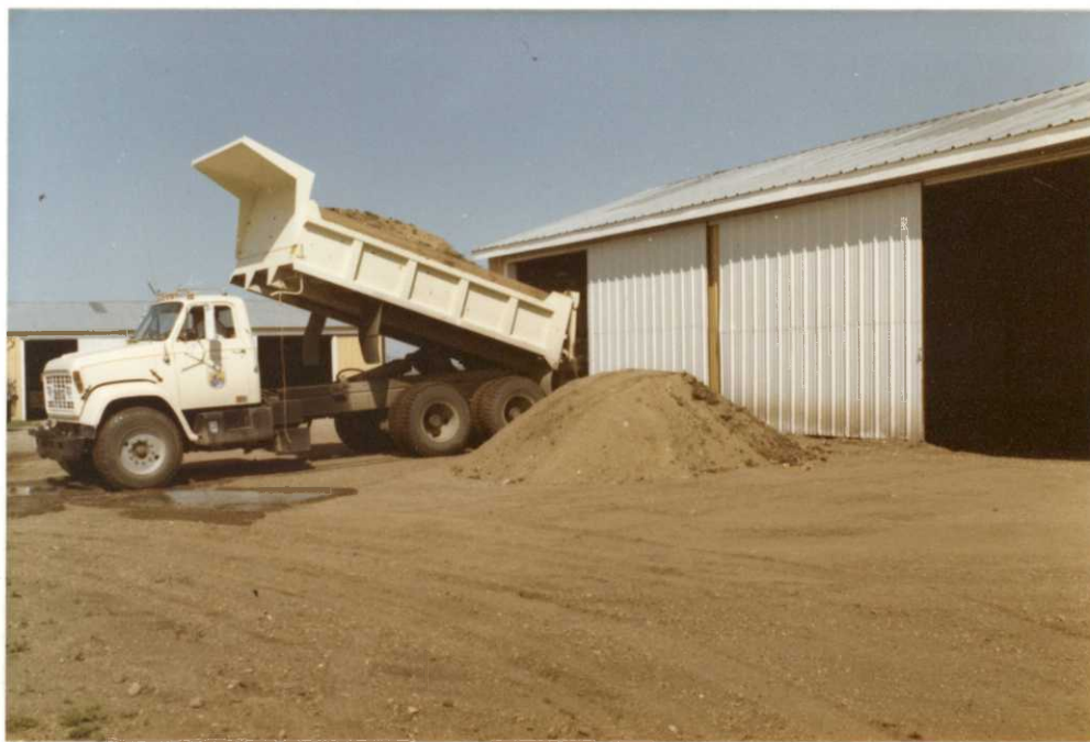
Photo 46. Arrowwood NWR graciously loaned us their modern equipment in order to accomplish site filling around our 30' x 60' pole barn, 7/84 - LDW.
