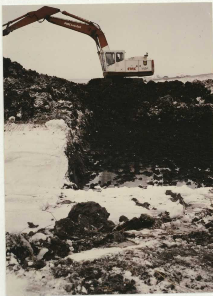
Photo 39. Construction was often difficult and messy when various natural springs were encountered during excavation of peninsula cut-off, note standing water at 10-15 o below temperatures, Brinkman WPA, 12/85 - RAH.
