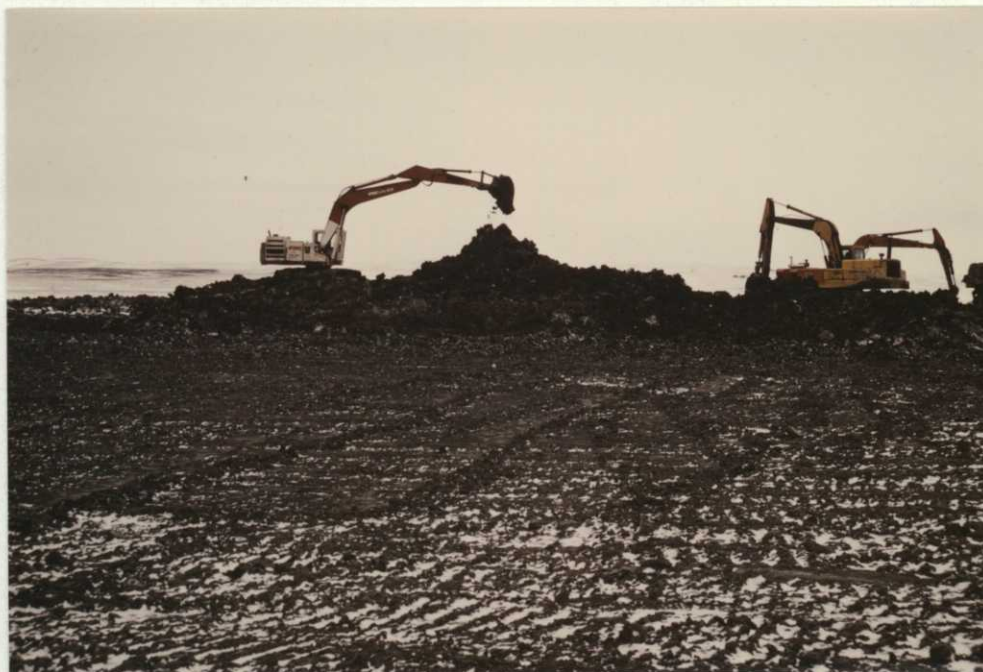
Photo 36. Ducks Unlimited (DU) contractor digging peninsula cut-off trench in frozen lake bed at the Brinkman WPA, 12/85 - RAH.
