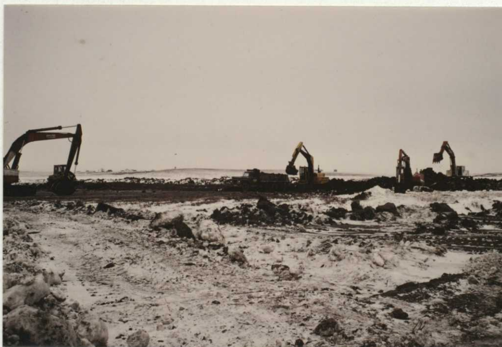
Photo 37. DU project with large selection of equipment digging trenches and filling trucks for nesting islands, Brinkman WPA, 12/85 - RAH
