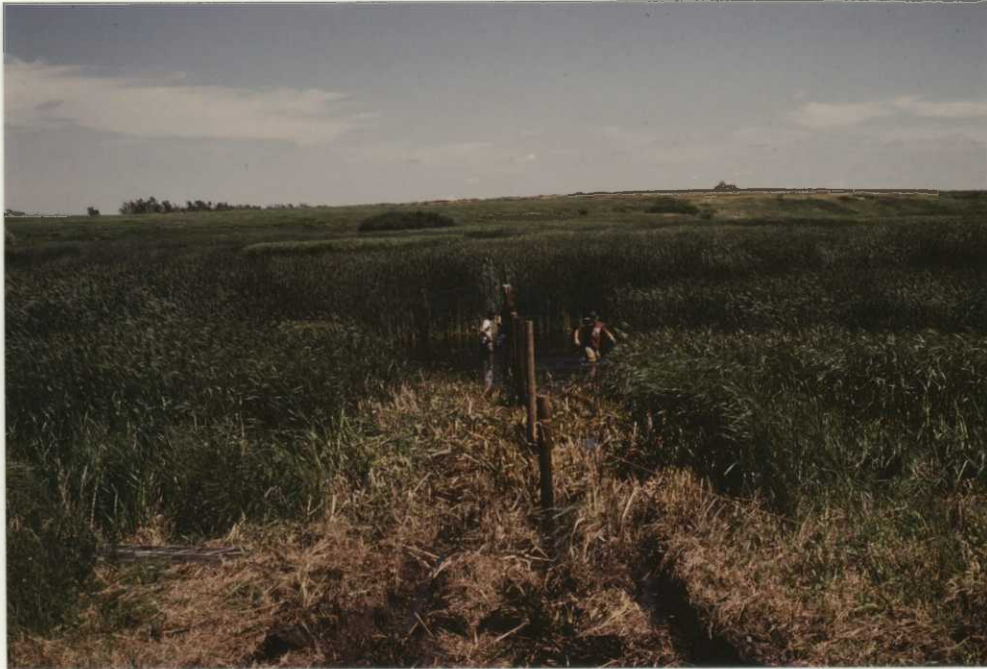
Photo 86-15. YCC crew building end of barrier. 60'-70' extension into water keeps most predators from moving around ends. 6/86-LDW.
