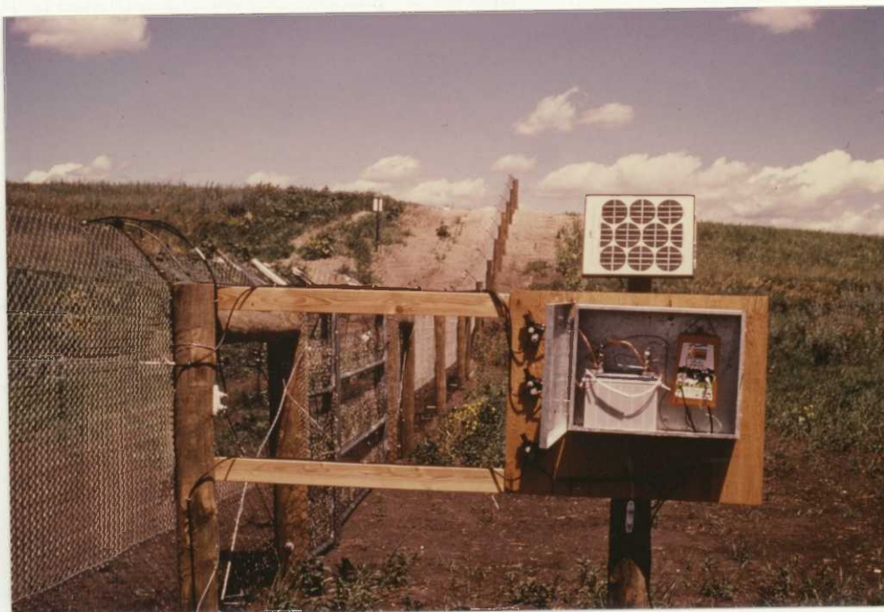
Photo 86-12A. Solar panel, powering an electric predator barrier fence.
