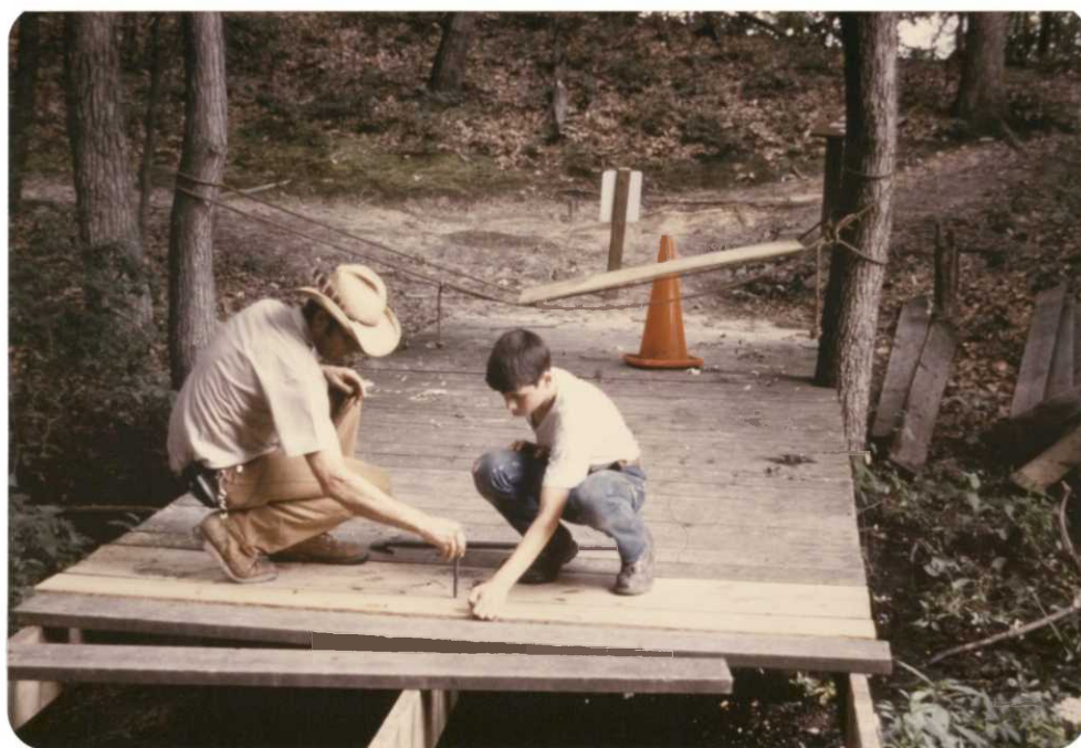
#3 Maintenceman Westerman shows enrollee Kenney how to space the boards on a foot bridge that the enrollees repaired. 8/84 YCC Enrollee
