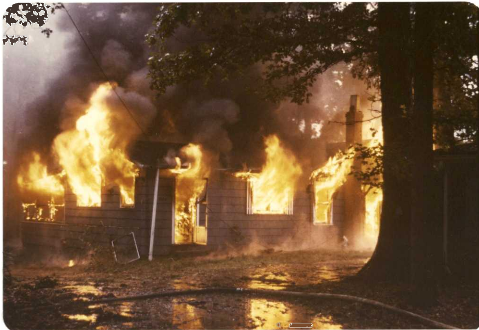
#19 The second building at Site 3 went with a hotter fire because it was still in good condition and almost air tight. 9/84 YMS
