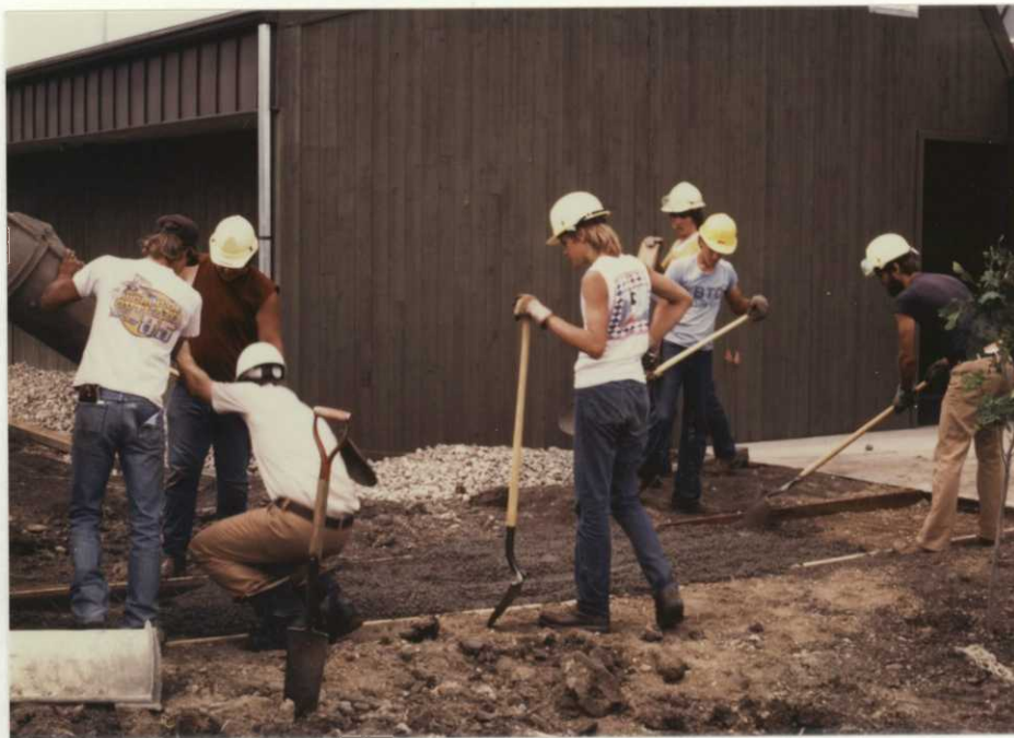
YCC crew pouring a new sidewalk at the office after installation of a new drain system. FGG.
