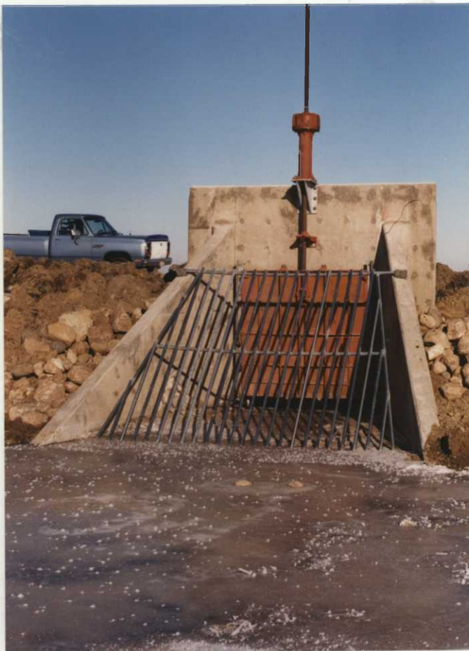
As part of Ducks Unlimited's Benson Unit Project, two 6-foot slide gates and new culverts were installed on the Upham-Willow City road. WLW.
