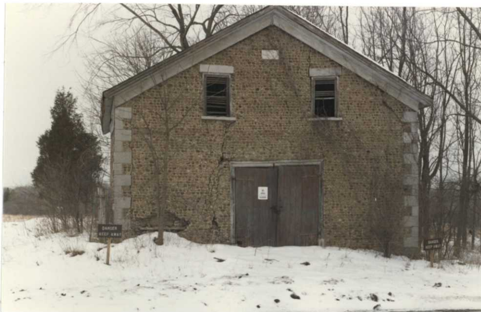
The Cobblestone Barn - an agreement reached with the New York State Commission of Historical Preservation may result in its removal during 1986. Both ends show severe deterioration; the sides are not much better (12/85; PEB).
