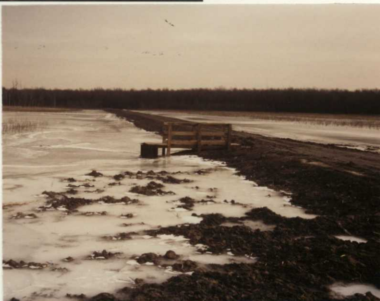
Completed Cross-dike Showing Stoplog Structure.
