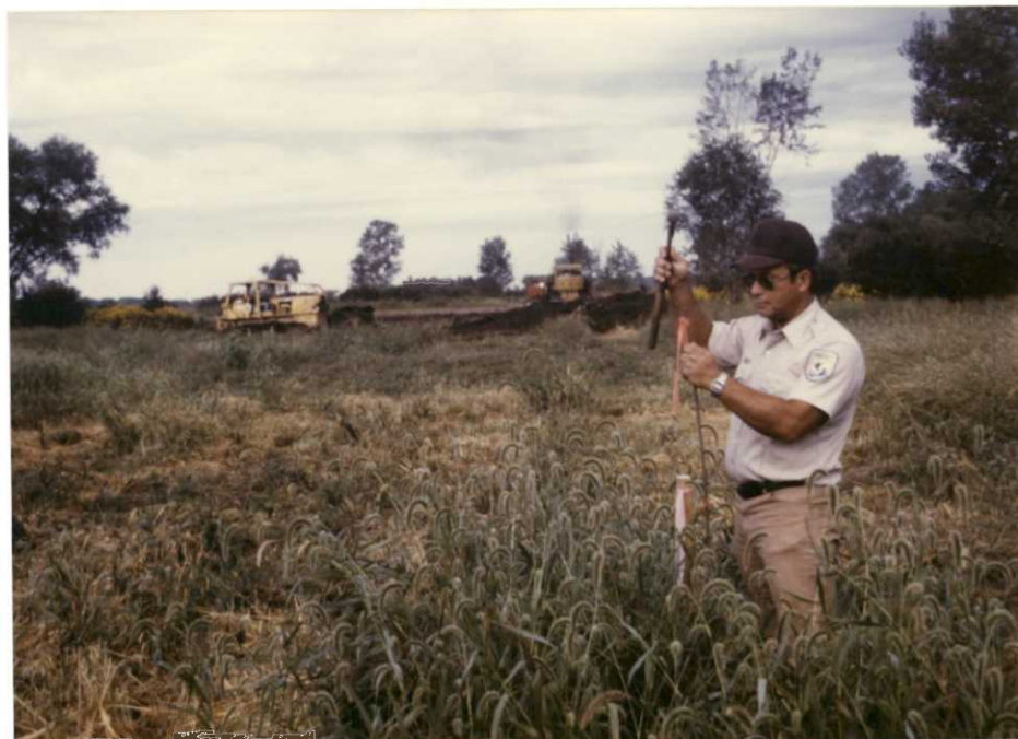
Chip sets a grade rod for a levee in the new moist soil units as dozers work in the background. BH 8/86
