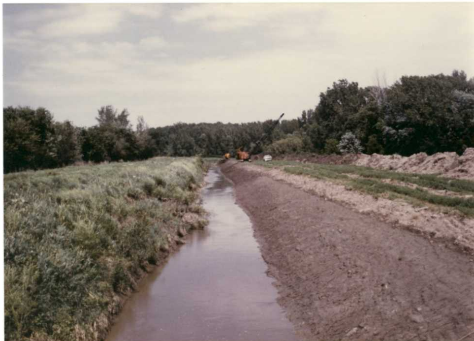
Two draglines clean the east side of Davis Creek ditch under an equipment rental contract. BH 8/86
