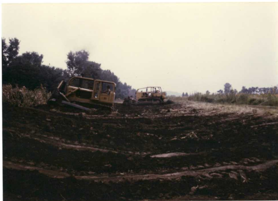
Two rented dozers build levees for new moist soil units. BH 9/86
