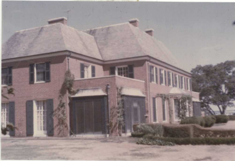
The mansion at Target Rock National Wildlife Refuge (TR-1-3, Gage)
