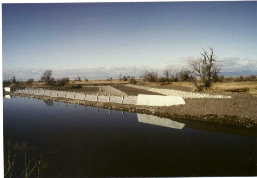
Bureau of Reclamation constructed emergency spillway near the end of the Closed Basin Channel.
