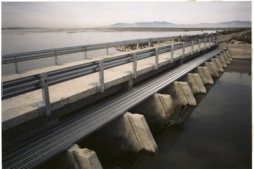
New catwalks and guardrails were installed on the spillways to improve safety.
