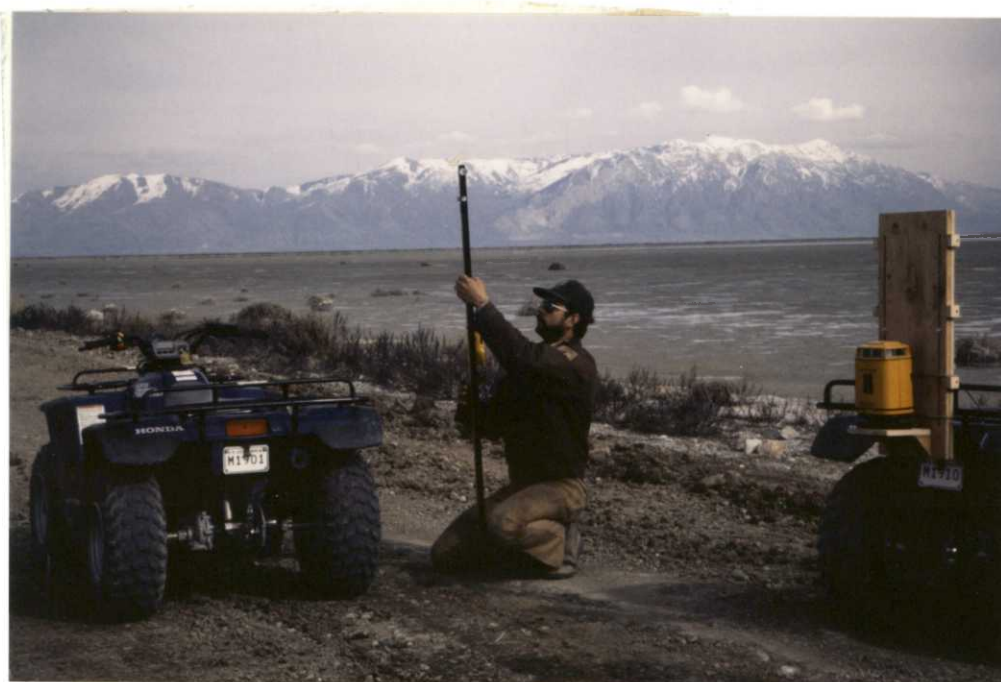
Equipment operator Iwanski adapted the laser level for use on the ATVs. Refuge dikes were then surveyed.
