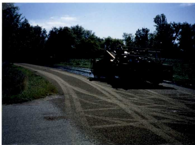
Figure 39. Major rehab work was completed on the auto tour route including bituminous overlay and/or seal coating.
