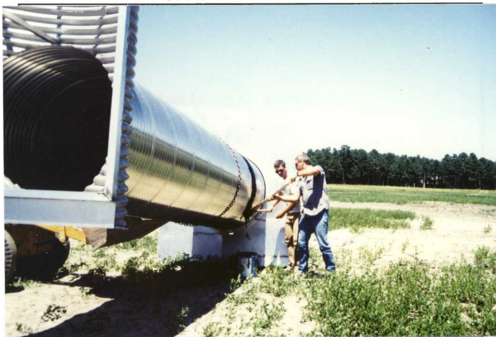
Fig. 114. Morris and Barker applying seep-shield to 72" diversion canal structure in Pool 5. (GAC)
