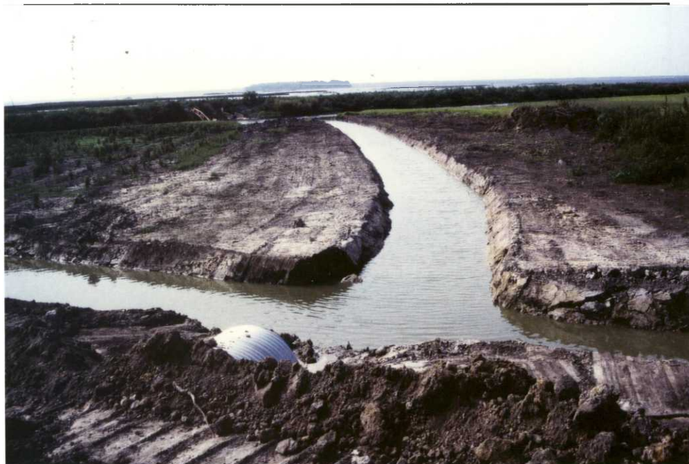
Fig. 117. Ditch excavated from 72" diversion canal structure to Wildlife Drive outlet structure. (GCH)
