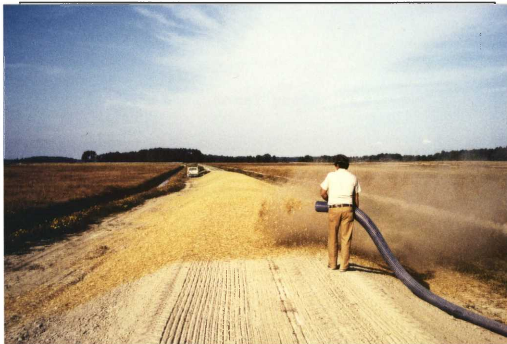
Fig. 122. All of the dikes were graded, seeded, mulched... (GCH)
