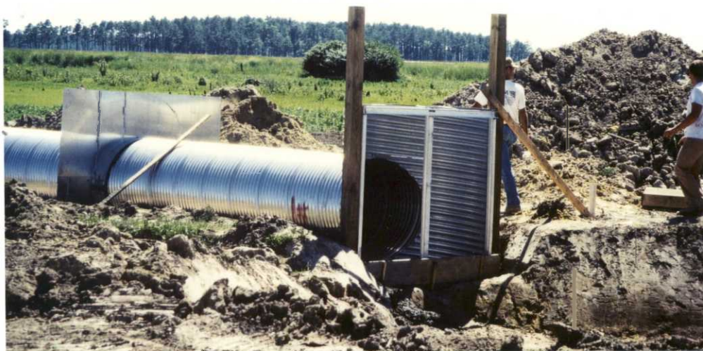
Fig. 115. Partially installed 72" diversion structure in Pool 5. (GAC)
