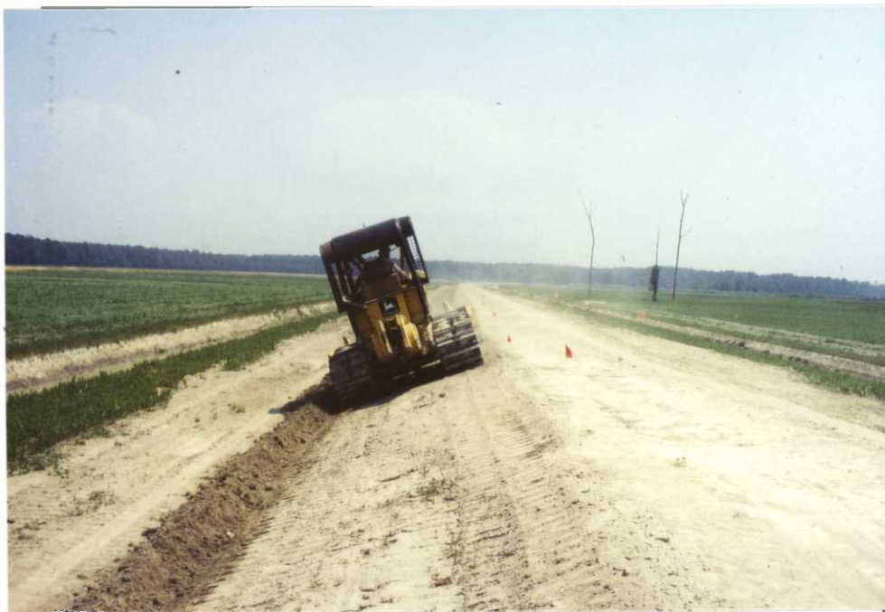
Fig. 121. The top width was established and 3:1 slopes cut with the dozer. (GAC)
