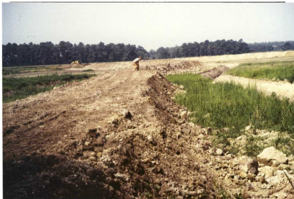
Fig. 120. Excavated materials were graded to establish rough elevations using the laserplane. (JAB)
