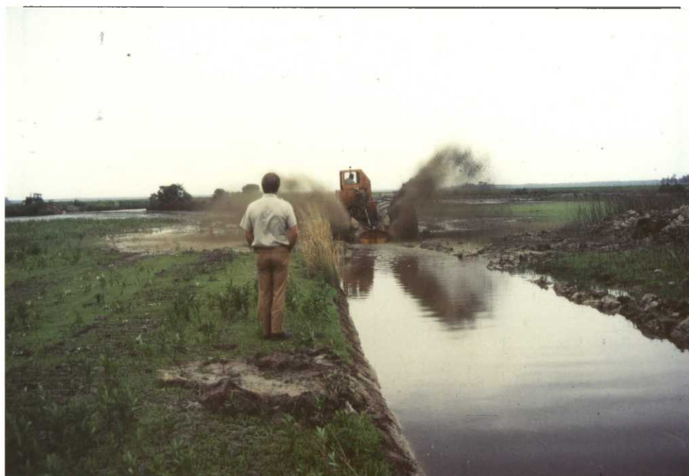
Fig. 48. Project Leader Carowan looks on as the GEMCO ditcher is used to construct a ditch to a water control structure at MSMU 5. (GCH)
