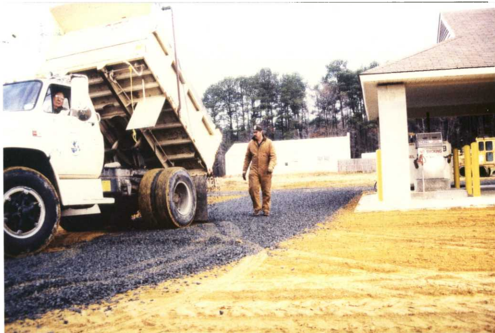
Fig. 101. 3/4" stone being spread dumped at new fuel storage building. (SLB)
