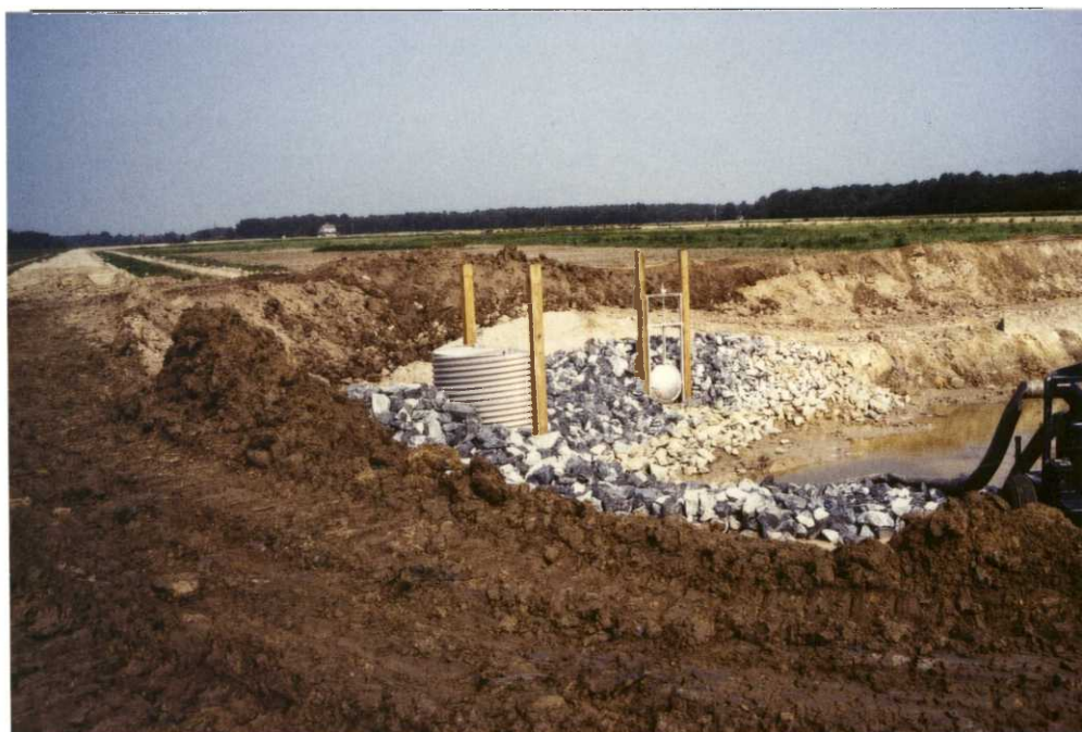
Fig. 116. Both 72" and 24" structures installed and rip-rapped at south end of Pool 5 diversion canal. (GAC)
