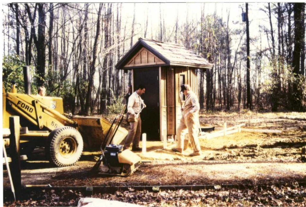
Fig. 103. ROS Barker and MM Webster constructed forms for concrete pad around new handicapped accessible toilet. (GCH)
