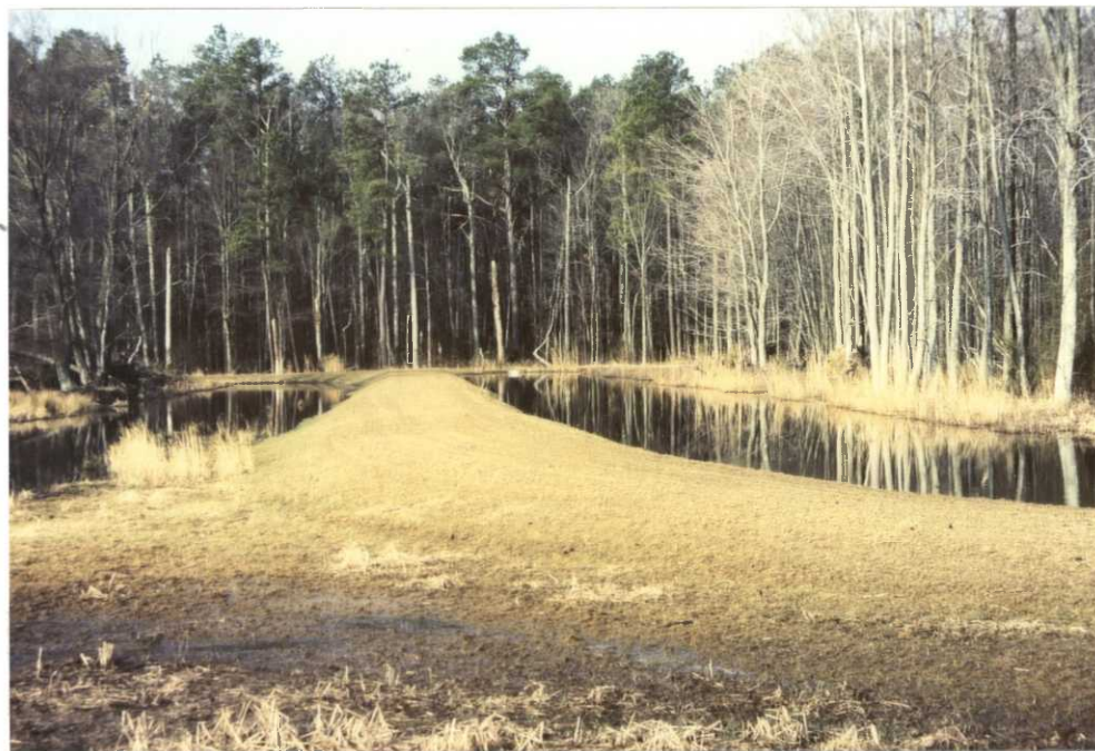
Fig. 110. Newly seeded dike that separates Pool 1 from Pool 2 GTR. (JAB)
