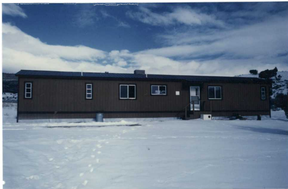
Quarters #115 after rehab. 11/01/90 Photo 29 TDO
