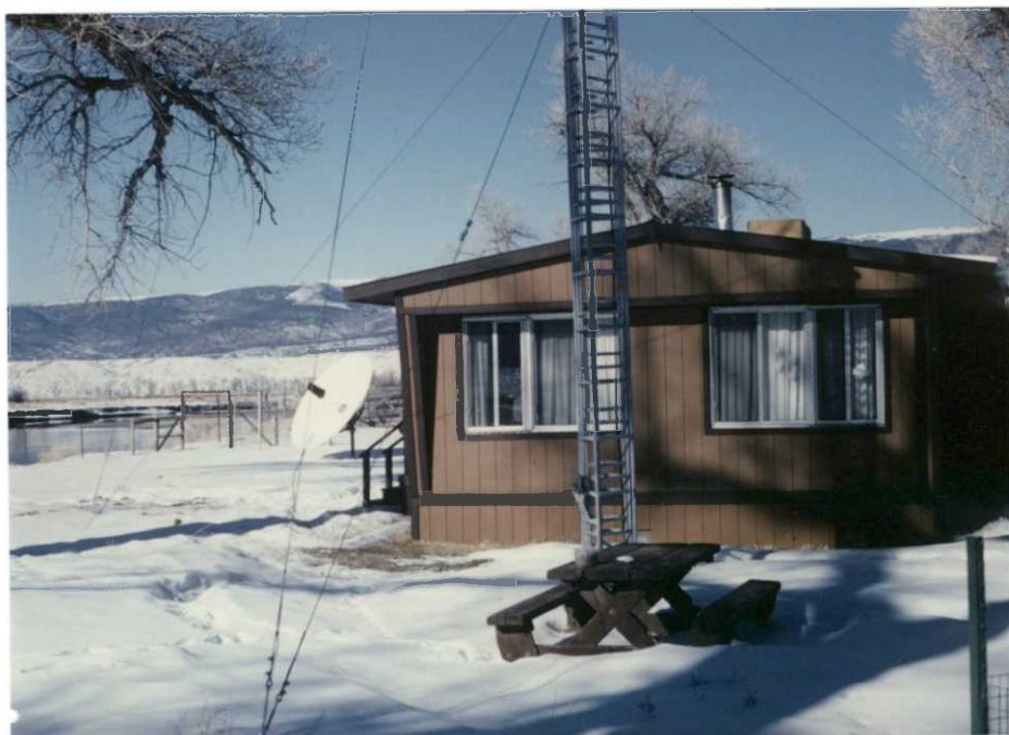
Quarters #114 after rehab. 04/30/90 Photo 27 TDO
