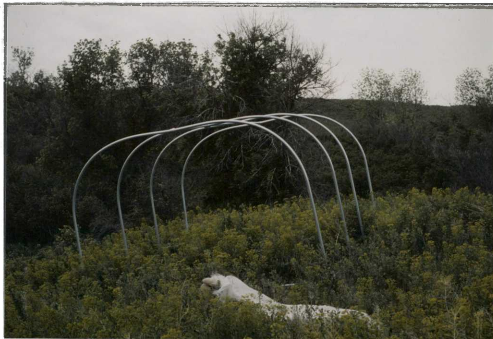
SUPPORTS IN PLACE. PTF
