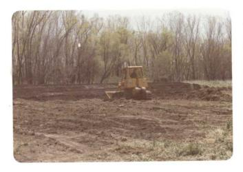
soils The appeared hydric, the vegetation was right, and the runoff above wet depression looked adequate, so a 150-foot gut plug, with tube and overflow-spillway, installed by forceaccount on the Thompson FmHA easement.
