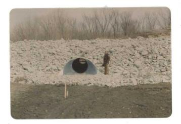
Iowa DNR engineered a 400-foot dike, with a 54-inch-bay Wisconsin structure. It was protected with filter fabric and 500 tons of rip rap. The \$30,000 project has the potential of impounding approximately 150 acres.
