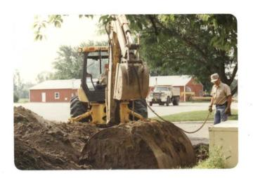
Two underground storage tanks at headquarters were removed by Evans Engineering the contracted amount of \$3,820. One served as the refuge station"; "gas other tank had abandoned when headquarters building switched from fuel oil to propane as a heatsource several years ago.9-4-90-12 RP
