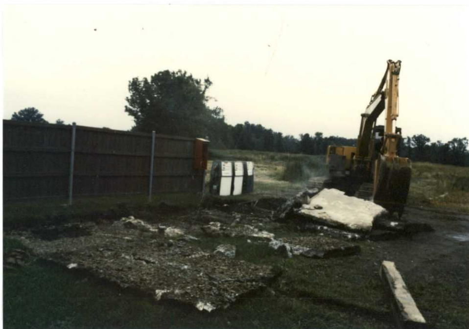
Contractor removing underground fuel tanks (TM)
