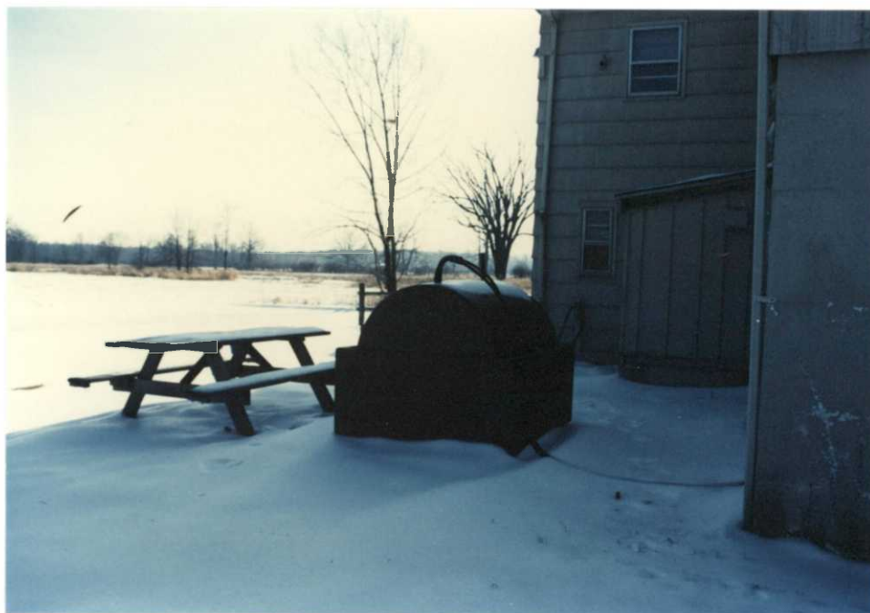
Above ground dike tanks replaced the buried heating oil tanks at Q-99 & Q-1; canopies still need to be erected (TM)
