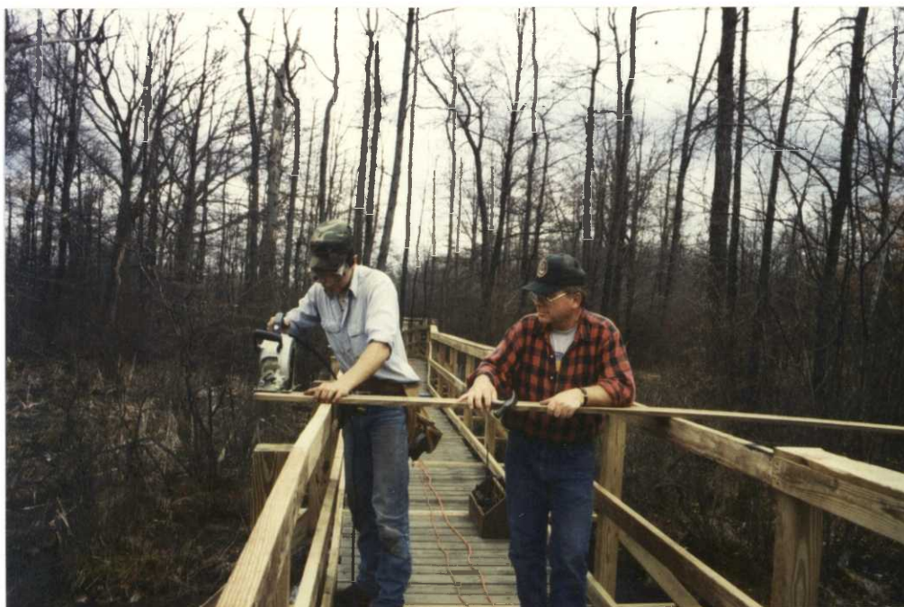
Laborer Balsamo and Volunteer Detizio adding handrails to elevated boardwalk. (TM)
