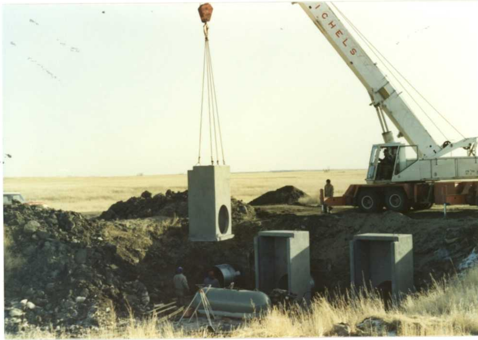
Figure 24. These vaults were hauled to Homestead and lowered into position. 11/91, DN
