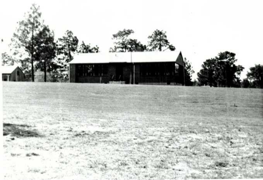
Quarters No. 4, front view after placing 1000 cubic yards of backfill to partially level for landscaping.
