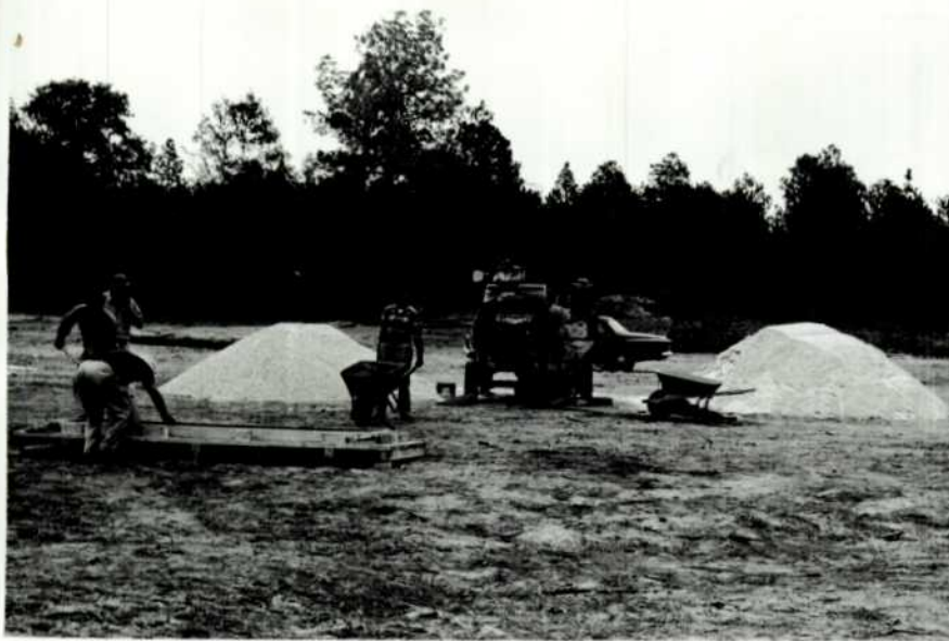
A concrete mixer was brought to the site, molds were built, and the tables were cast.
