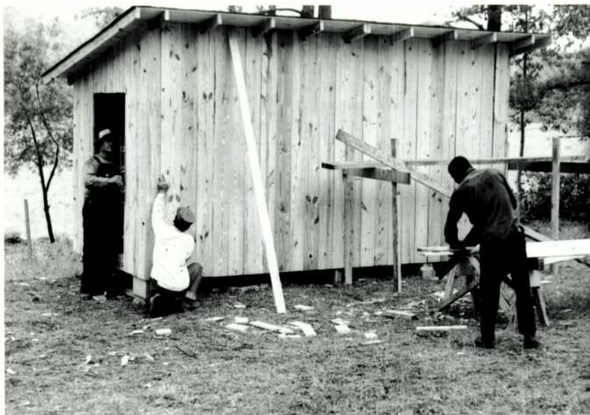
A temporary tool and materials shed is prefabricated by APW crew at field work station.
