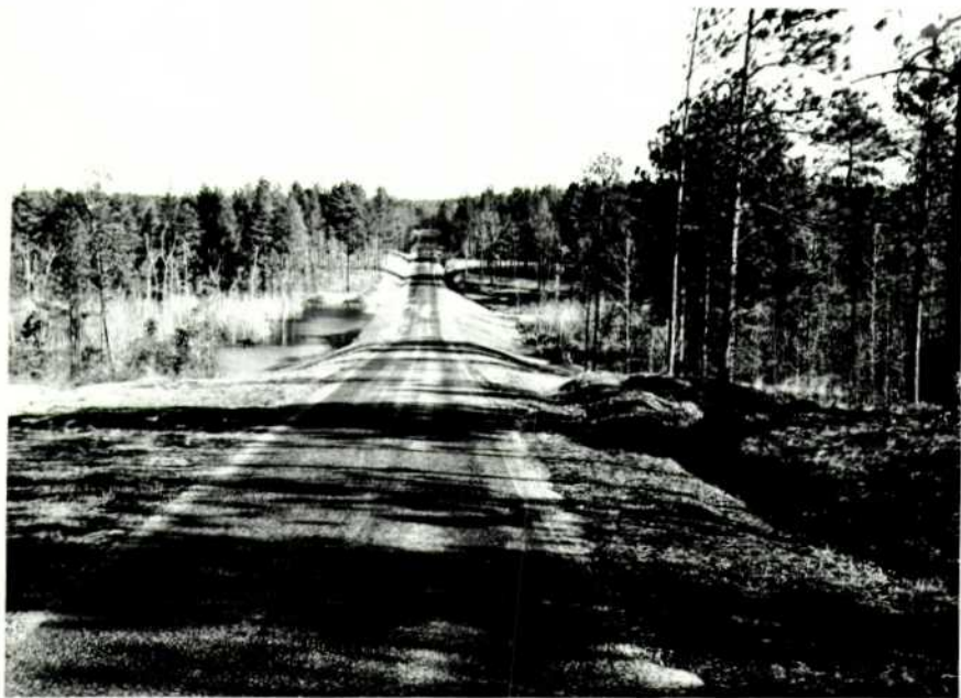
Road work complete. This fill on Ham Branch at the head of Martin Lake impounds 29 acres of water which will be managed as a green-tree reservoir. No. 13
