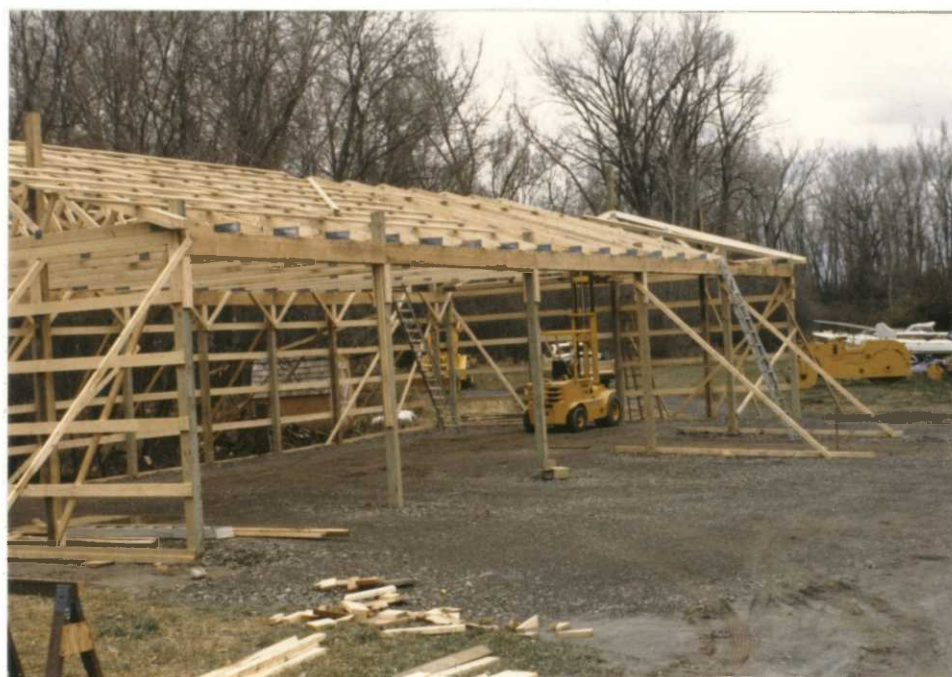
The refuge's new open-sided pole barn being built (88-9; KAJ).
