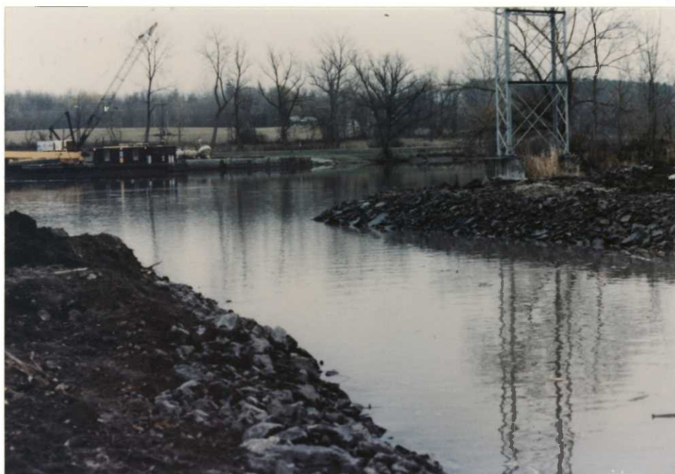
Channel opening into the north end of Cayuga Lake showing intermediate rip rap as slope protection. The barge in the background was part of a neighboring State construction project (91-26; SLF).
