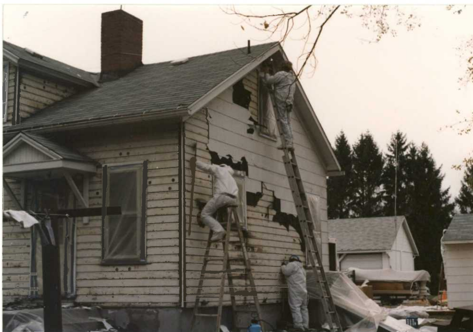
Removal of the asbestos siding from the refuge quarters (91-28; MJN).
