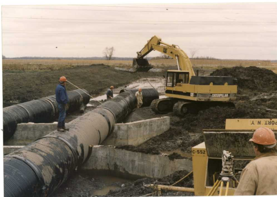
Setting the final pipes which will carry the water over the second of two ditches draining the northeast section of Unit 17 (91-24; SLF).
