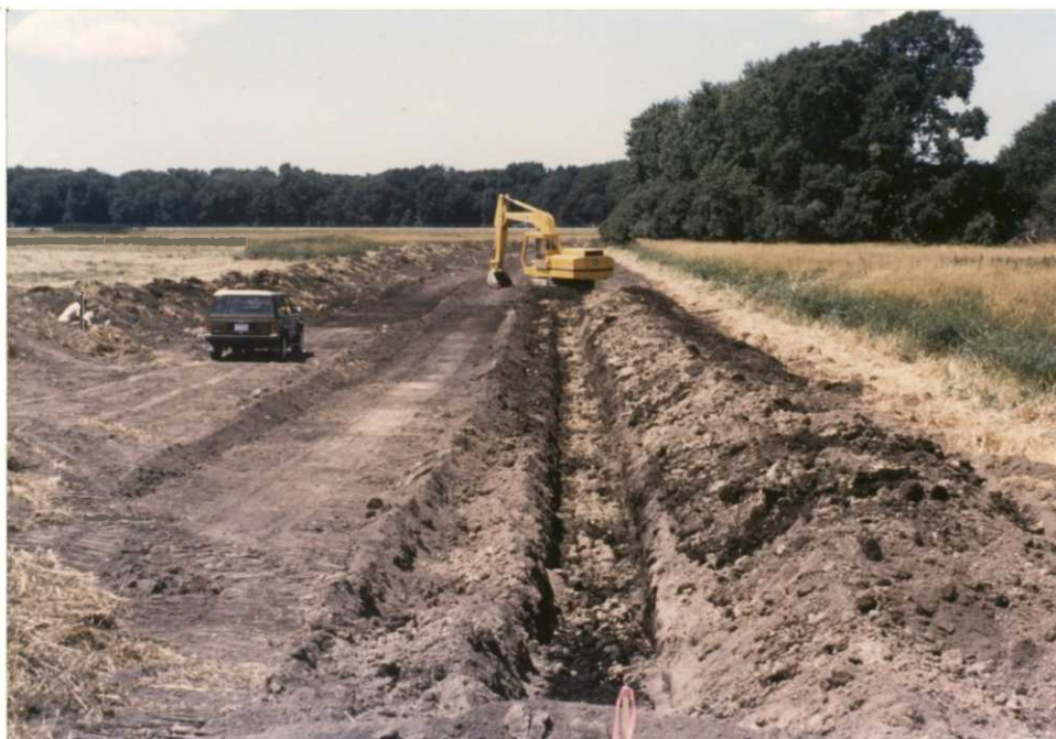
Excavation of the core for the Benning Marsh Dike. Marl for the core (good clay was not available) was borrowed from the area to the left of the trench (91-27; TAG).
