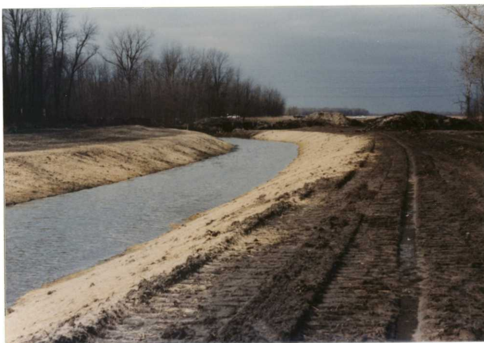
Finished channel showing approach to the North Dike area. Slopes were hydroseeded late in the year, but unseasonably mild weather prevailed and good germination resulted in most areas (91-25; SLF).
