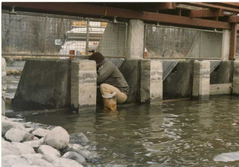
Maintenance Mechanic Flanders installs the new aluminum carp control grates in the White Brook Spillway (91-30; BLC).
