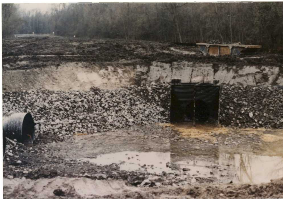
North side of the Unit 17 South Dike showing pipes under the South Dike and the water control structure feeding or draining the Unit 17 southeast drainage ditch. Background shows use of the South Dike for excess spoil deposition (91-22; SLF).
