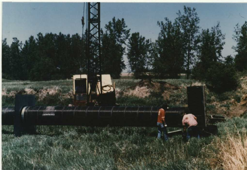
Contractor installing stop log structure on Moen WPA, Pope County. 6/2/88 BLA 88-37
