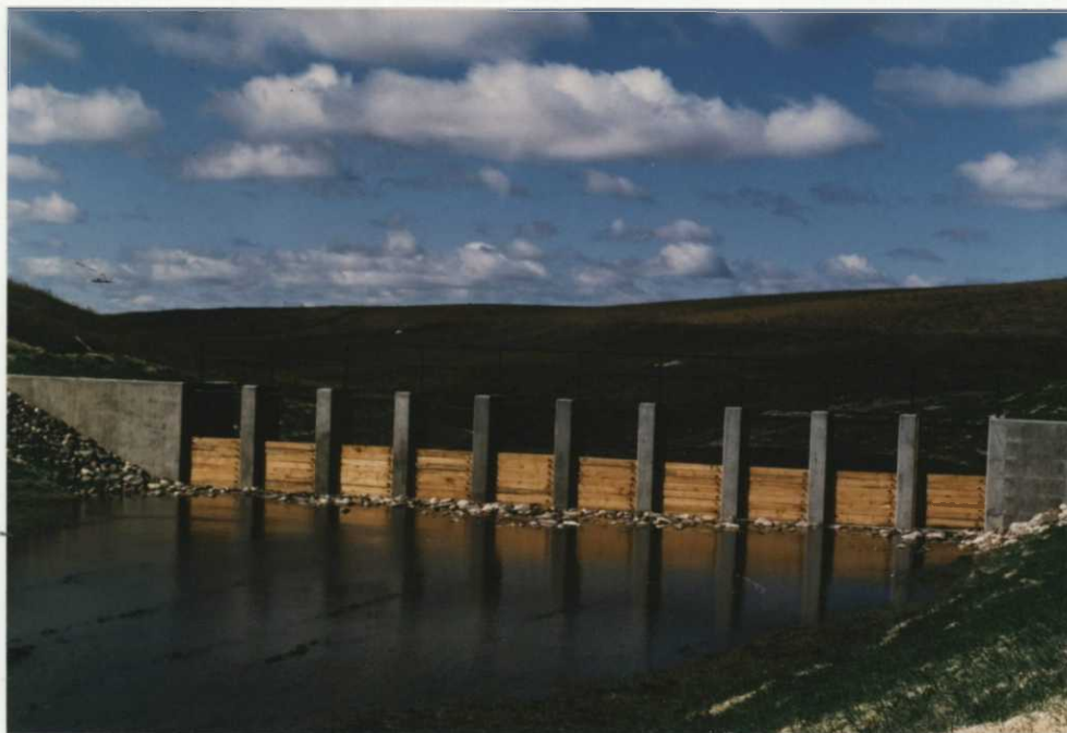
Structure I. The lowest structure on the watershed and lack of emergency spillway site, resulted in a structure with 50 feet width of effective boards for spillway and water level control. 10/2/88 BLA 88-35
