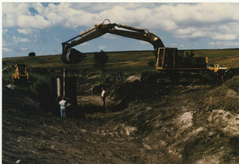
Contractor setting one of two full round risers that make up Structure H. 7/20/88 BLA 88-36
