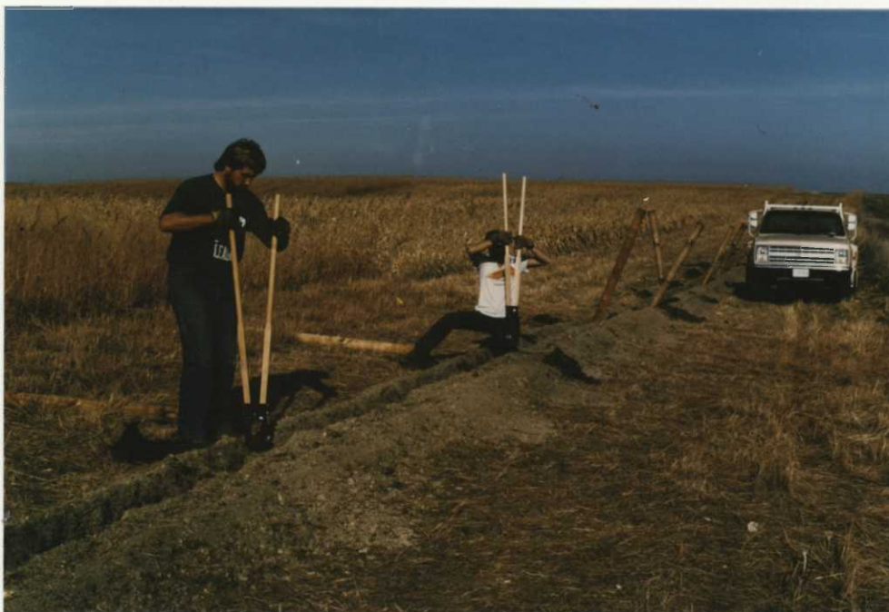
Temporary Biological Aids digging post holes and setting wood posts for predator exclosure. 11/1/88 FLA 88-40
