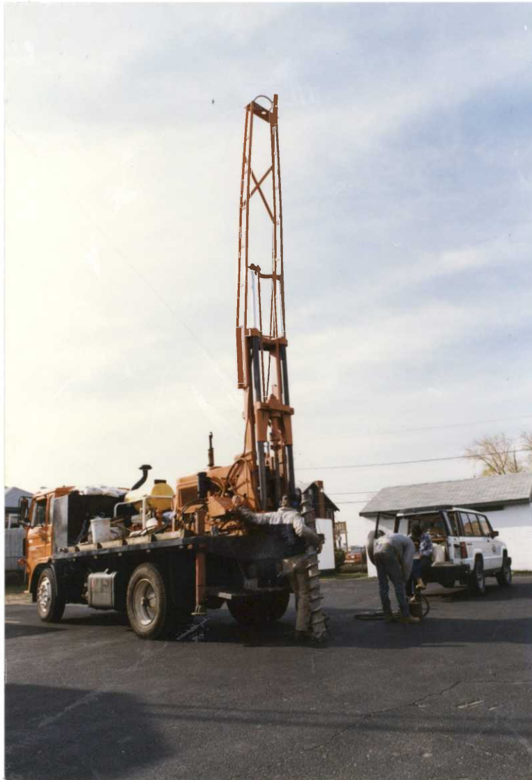
Contractor installing monitoring well; part of a process to ensure groundwater at refuge headquarters is not contaminated by leaking gasoline tank.
