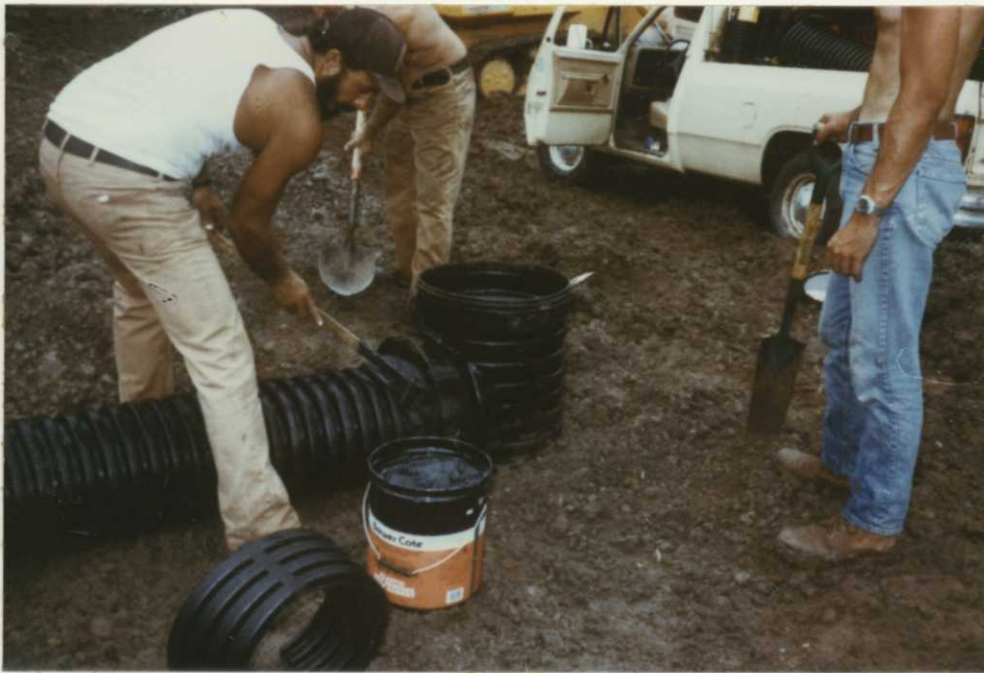
Work often included installing a drainage culvert with riser. We normally made use of the common plastic culvert materials. (SC)
