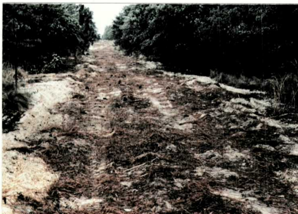
June, Area 3. Grass seed was drilled and the area mulched with pine straw by hand. (88NR-39, 6-88, Cartlidge)
