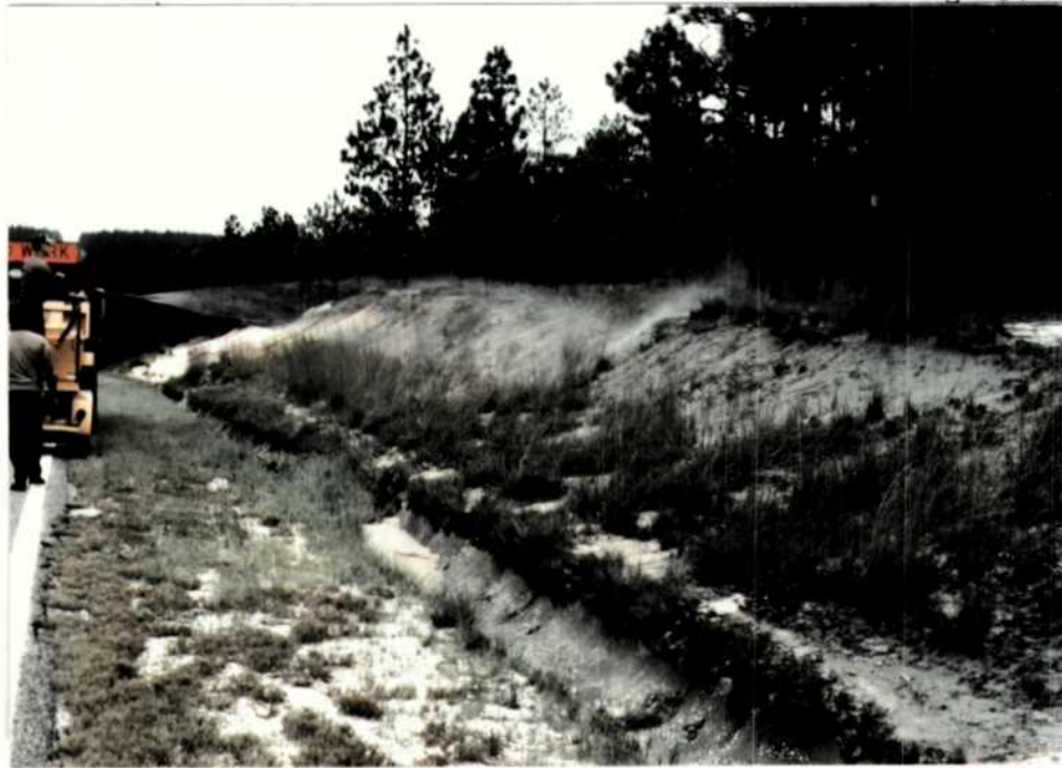
The highway department applying a mixture of grass seed and fertilizer with their hydroseeder. (88NR-30, 9-88, Cartlidge)
