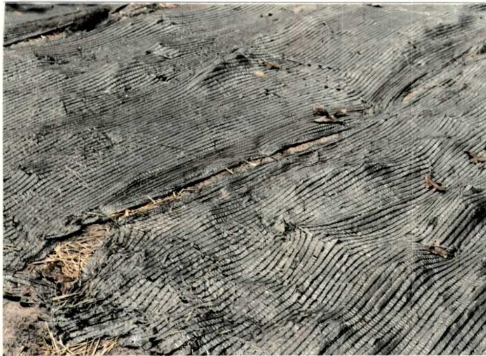
June, Area 2. Grass seed was drilled and the area covered with a paper/fiber type erosion control mat. (88NR-36, 6-88, Cartlidge)
