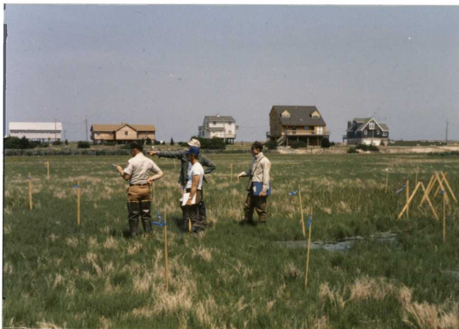
Refuge and ES personnel meet with State Biologists on-site prior to excavation of each OMWM area. This area adjacent to Broadkill Beach, was completed by November. The stakes indicate ditches, sill and pond locations.
