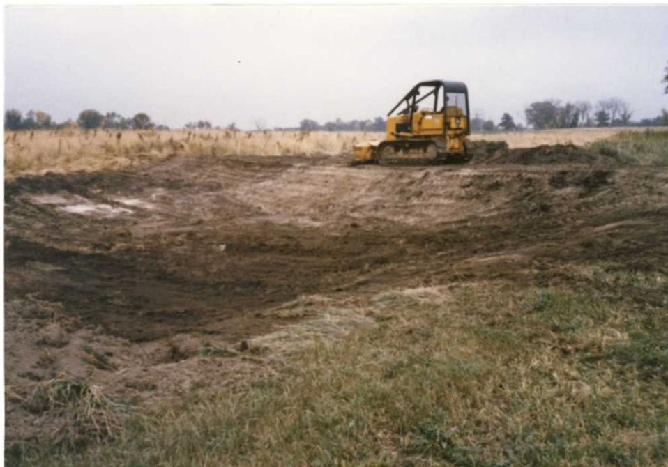
Wetland restoration on private lands comprised a major portion of Sherburne's program in 1988. Both photos were taken on private lands in Isanti County, MN. A dike starts taking shape in the above photo and the finished product on the James Nyman farm below. (AWR & BDE 8/88)
