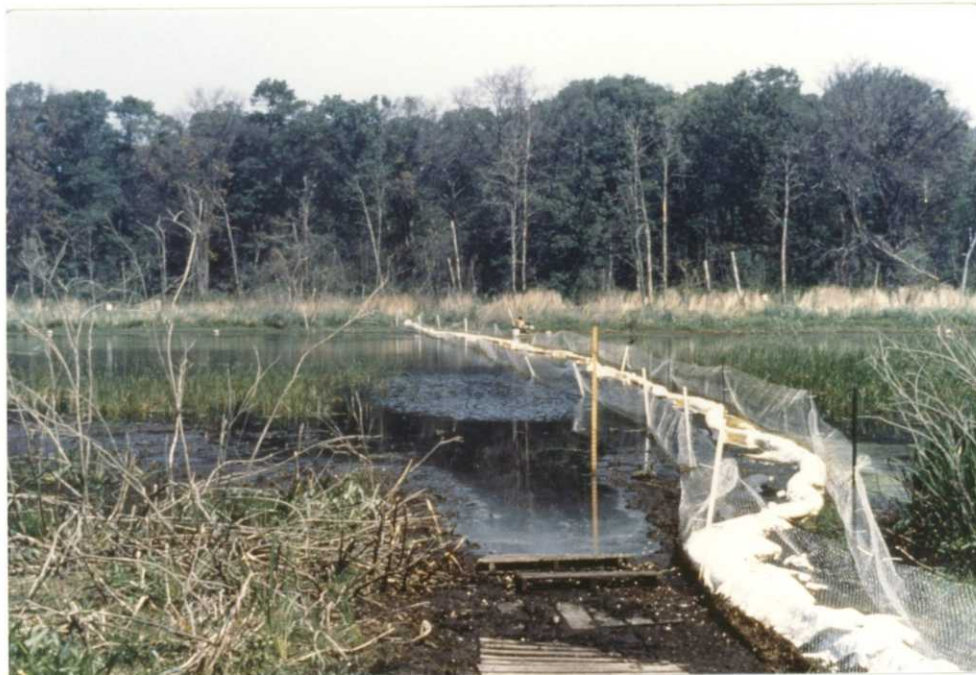
A methoprene-impermeable barrier was installed in each study marsh. (University of MN photo - 1988)
