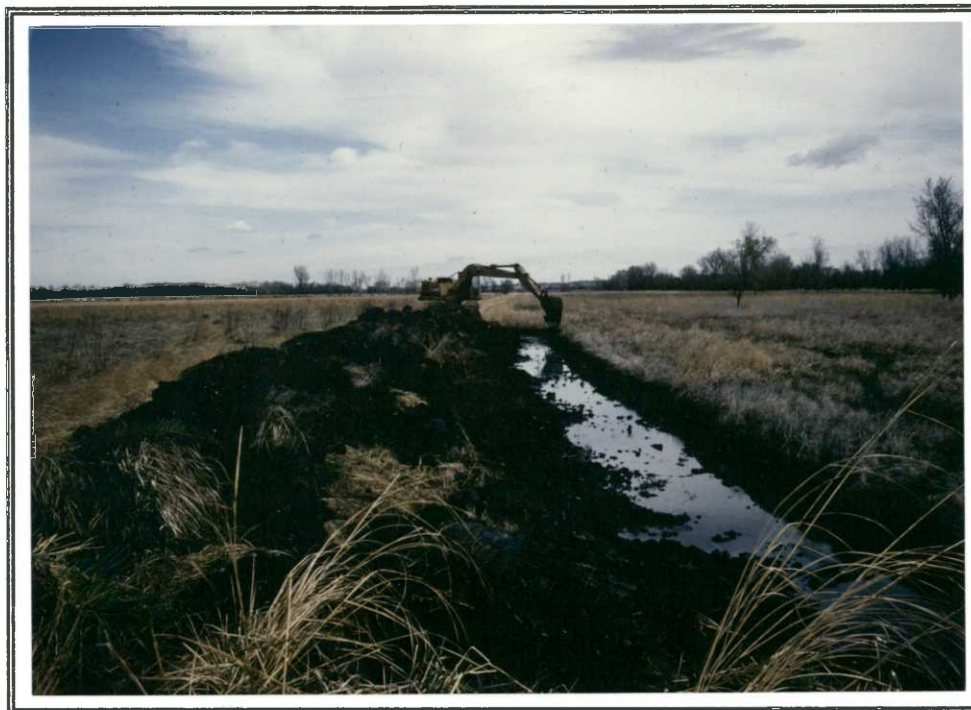
A tracked excavator was used to rehabilitate the Rice Paddies Moist Soil Unit ditches. 4/91 RLB
