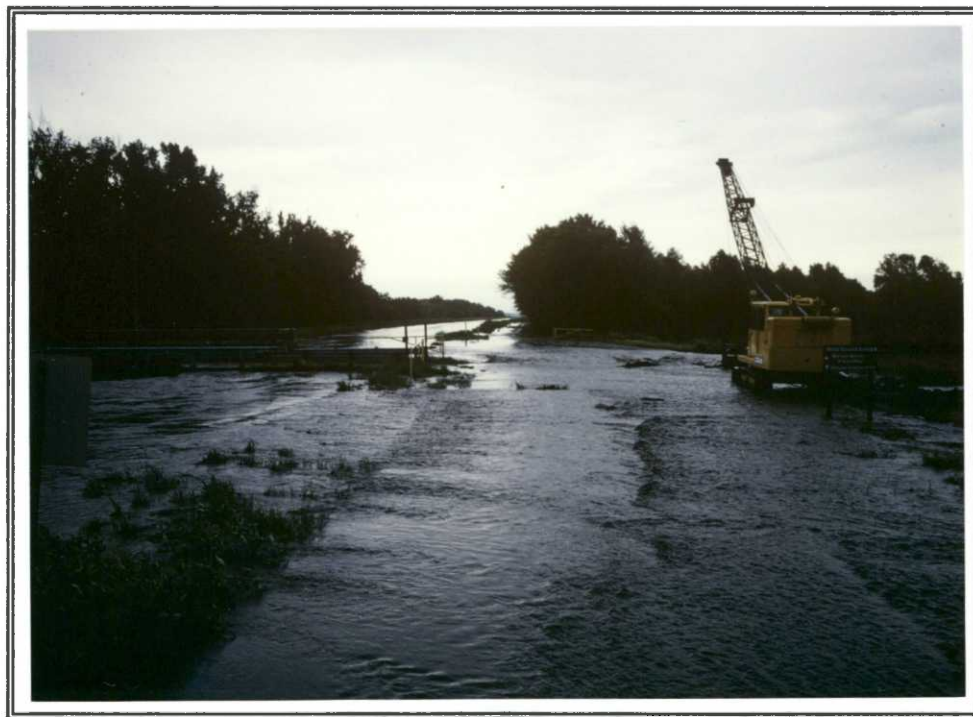
The ground under the dragline nearly washed away in the July storm. 7/91 RLB
