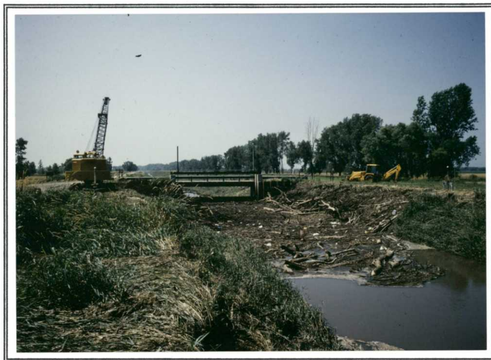
A large volume of trash and debris collected around the water control structure after the late June flood. A dragline had to be used to clean up. 6/91 RLB
