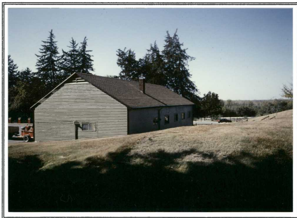
A new furnace was installed, heated section insulated, new shingles added and entire building painted to match the new shop. 10/91 RLB
