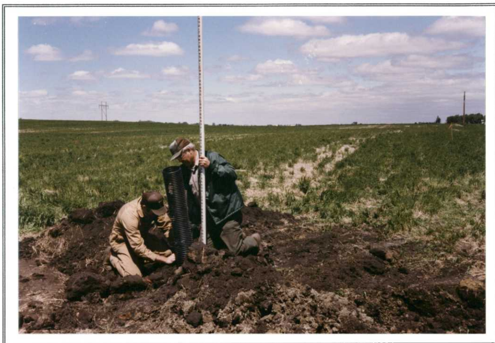
#14 - Wetland restoration activities may involve both removing or installing drainage tile. (DT, 5/90)
