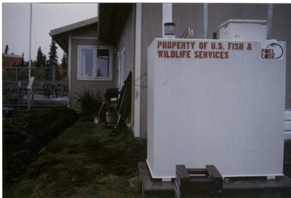
Residence No. 28's leaking fuel line. The break was at the right angle under the window. 09/26/96, RDP
