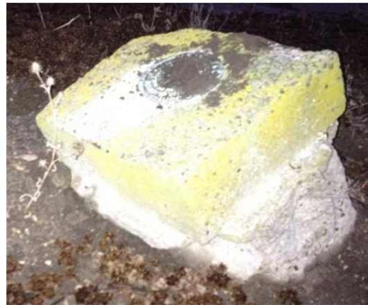
Picture 2. Destroyed benchmark located on Naval Weapons Station Seal Beach
