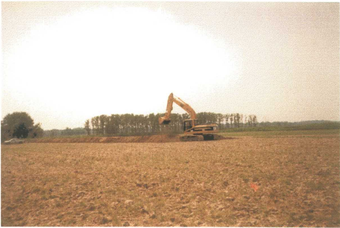
Here the State operator with excavator is proceeding east with construction of the north levee.
