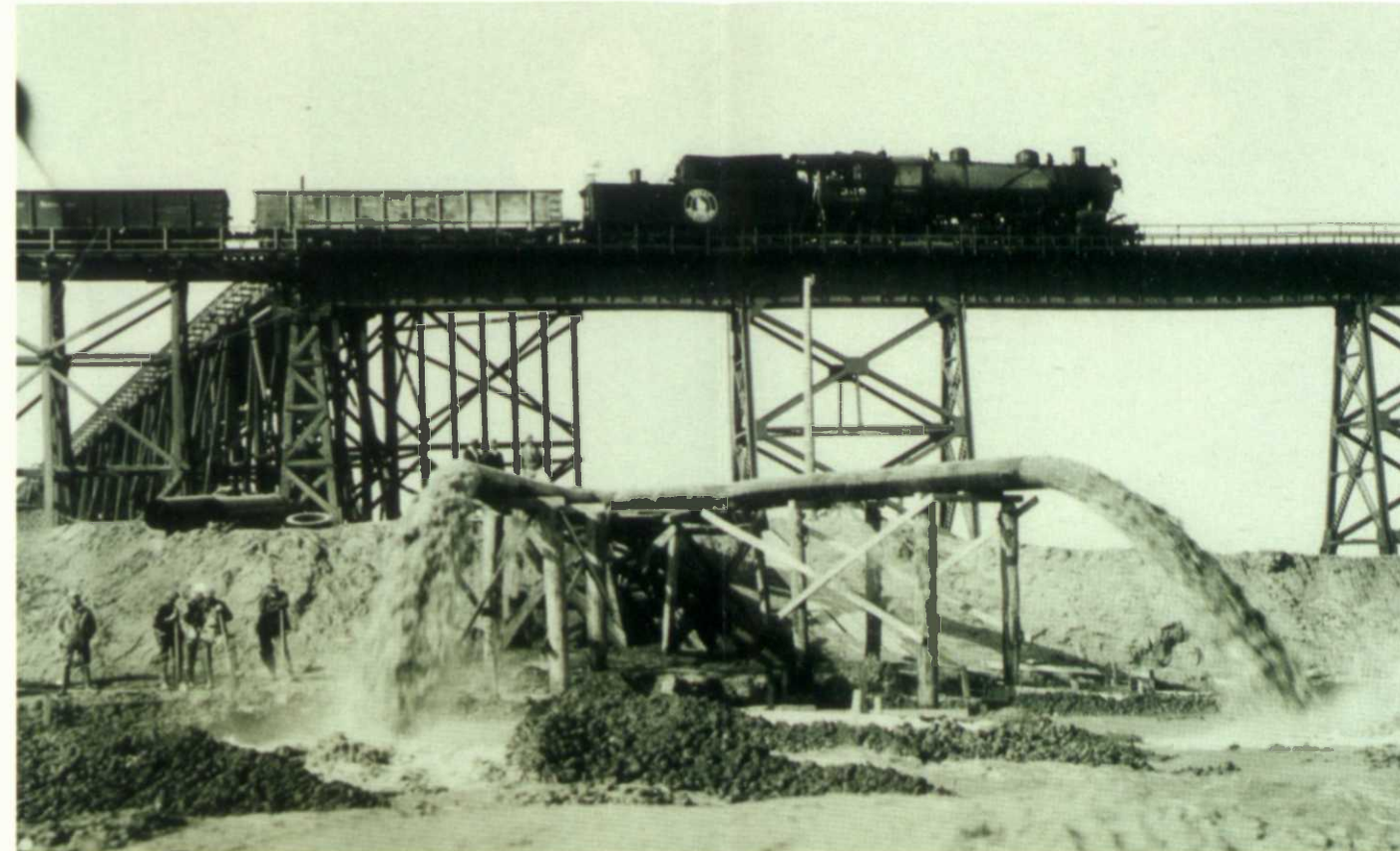
Dredge pipes deliver slurry to the core pool as a train loaded with rock and gravel passes overhead. When the water drained out of the core pool, clay and impervious soils remained to form the core of the dam. The rail bridge is now entombed inside the huge Fort Peck Dam.
