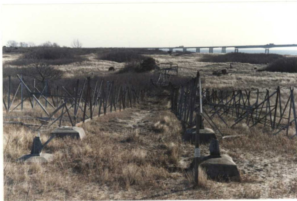
LH 1987 After: The tower has been cut in half and laid on it's sides. The Navy successfully cut-up four out of seven towers.
