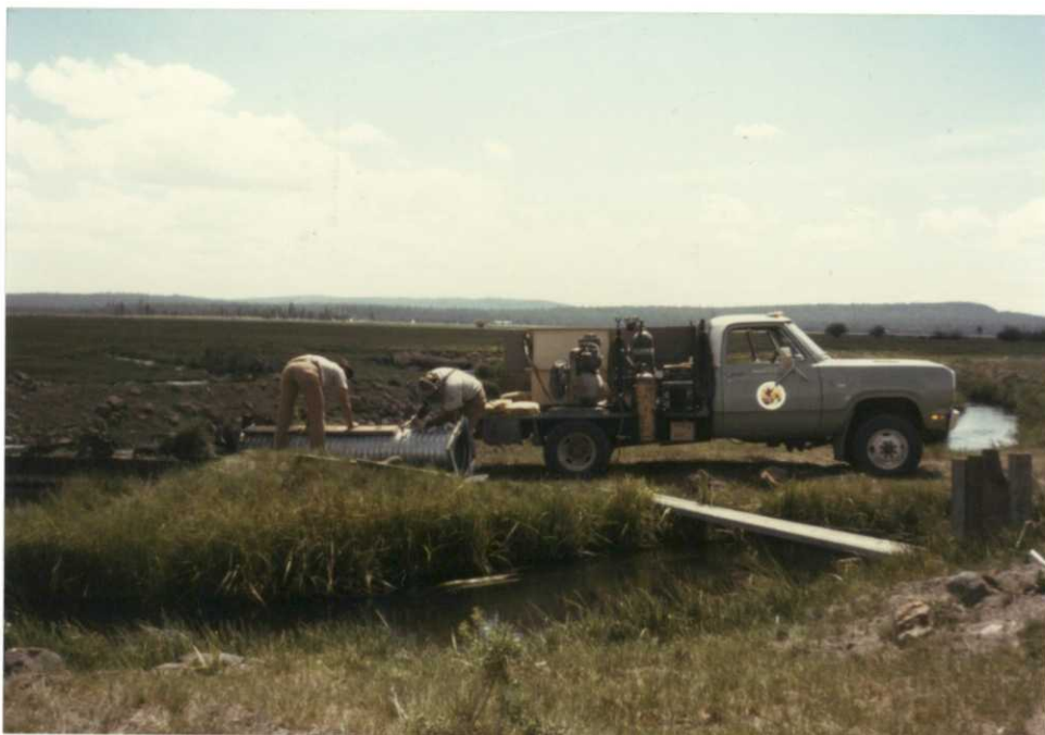
KM-90-12 Cole, Moore installing water gauge recording station below headquarters. DL 7/90
